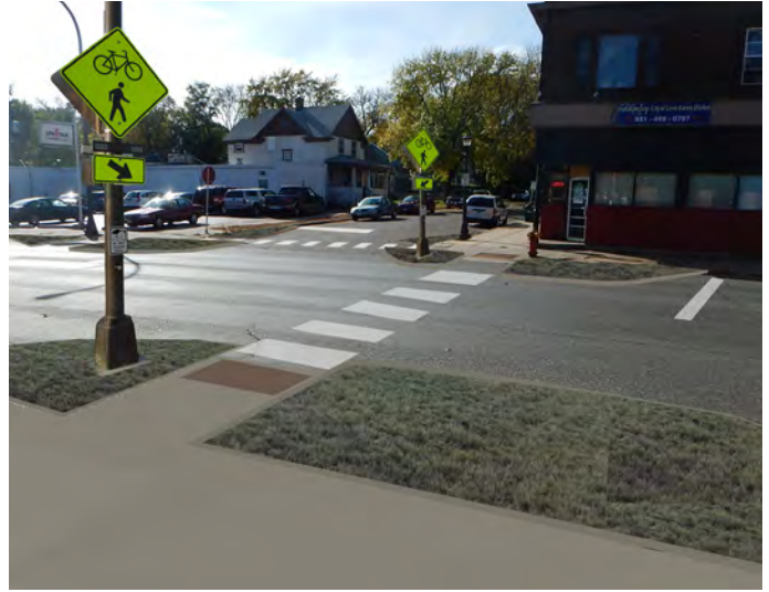
Recommendation B. Intersection of Jenks Ave and Arcade St. Current (left) and recommended (right). These improvements would make the crossing distance shorter and would bring more visibility to pedestrians.
