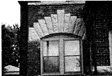
Typical masonry details used on historic Dayton's Bluff residential buildings. Any repair or replacement should match the color, texture, and detail of the original material.
