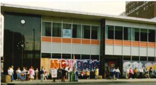
Figure 2.9 An example of mid-century modern architecture near the Central Station site in Saint Paul exhibits many of the common characteristics including an “industrial” look as well as a metal and glass skin.
