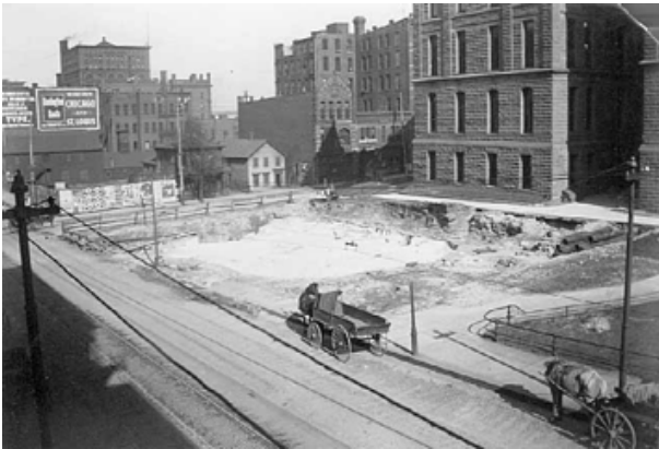
Figure 2.2 View of 5th and Cedar corner, Central Station block at rear. ca. 1900
