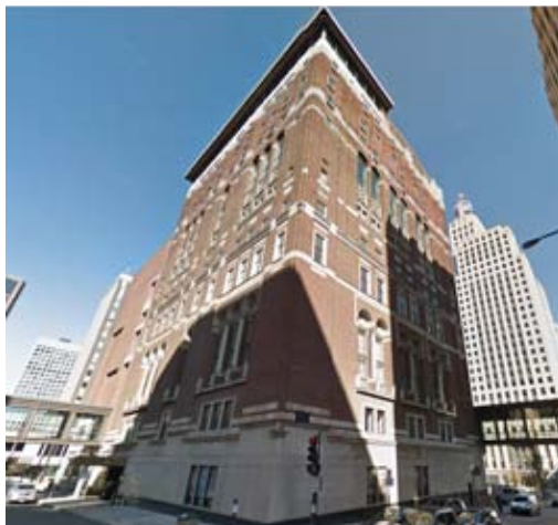
Figure 2.17: The Saint Paul Athletic Club occupies the southern corner of the Central Station block; Google, 2016
