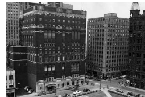
Figure 2.23 The Minnesota Building, in the middle
