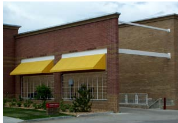
Figure 5.12 Consider screening service equipment or areas using materials and designs that are compatible with the new development(s).
