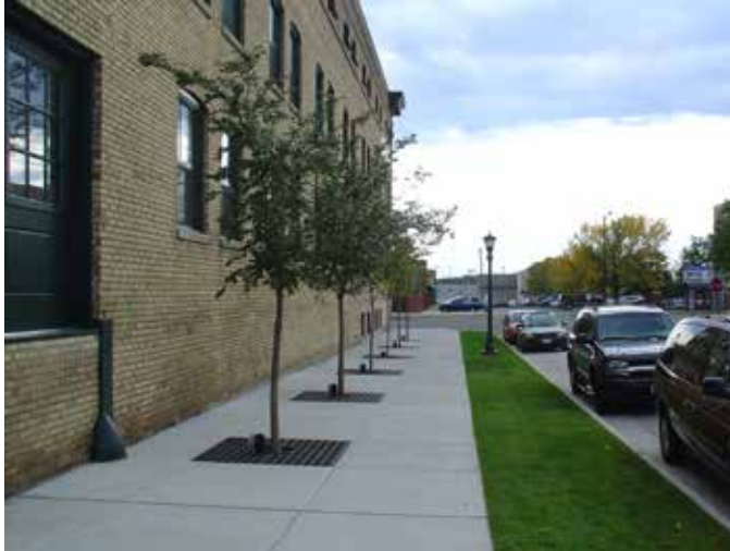
New sidewalk and streetscape on Carleton Street
