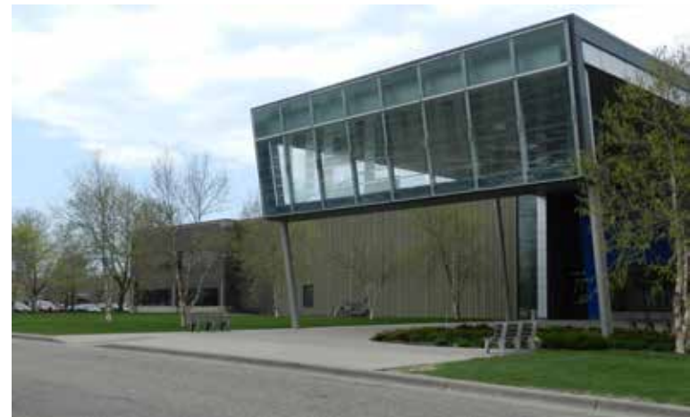
University Enterprise Lab (UEL) located in the Westgate Area
