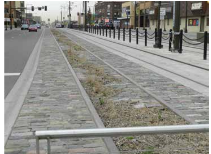
Green Line LRT tracks on University Avenue
