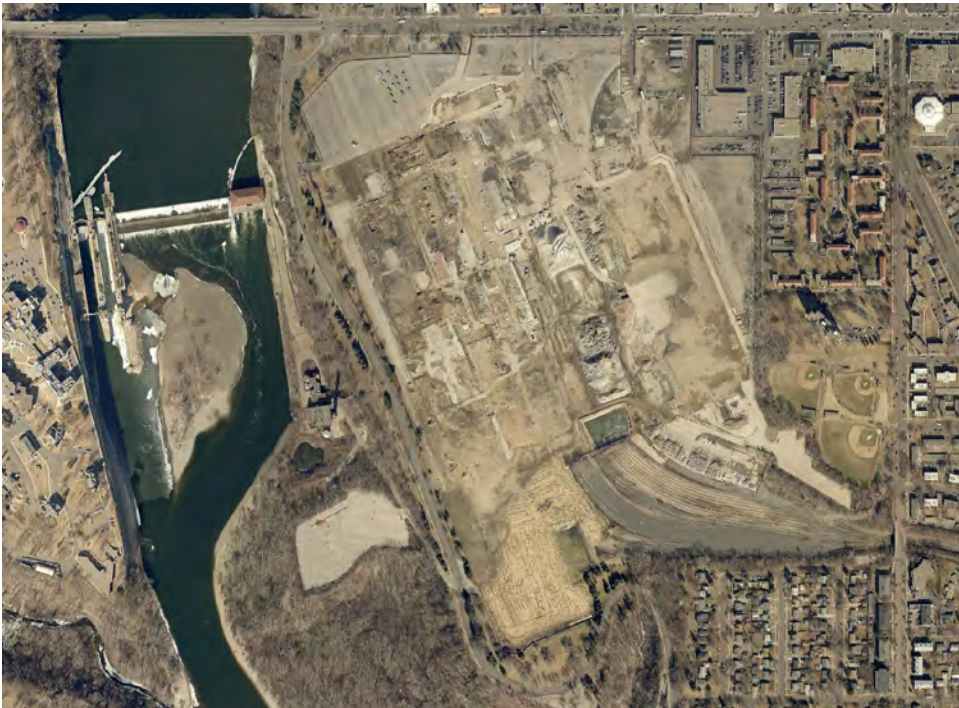
Ford site demolition 2015.
