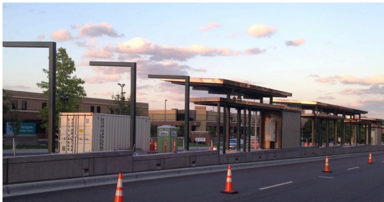
Future Westgate Light Rail Station, St. Paul
