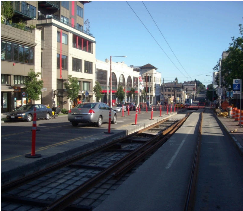
First Hill Streetcar construction, Seattle
