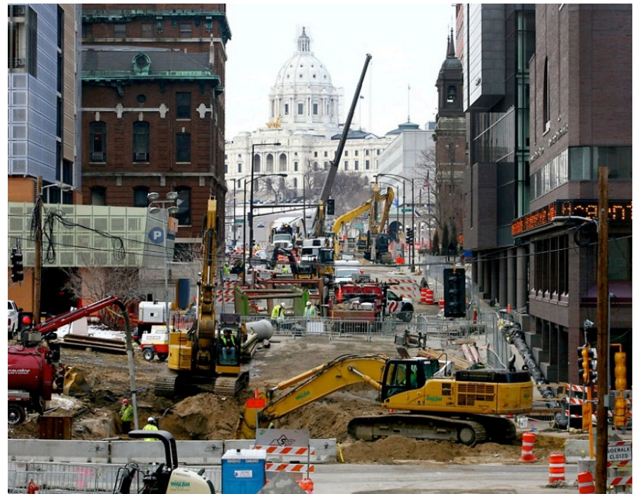
Green Line construction, St. Paul
