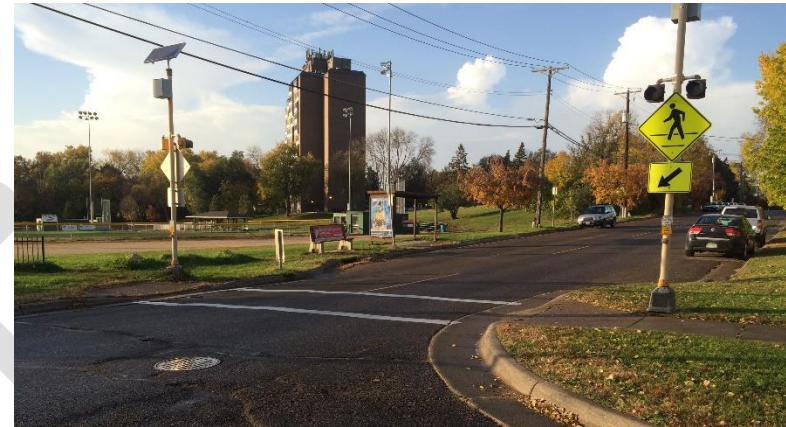
Figure 2-12: Missing sidewalk alongside Cleveland
