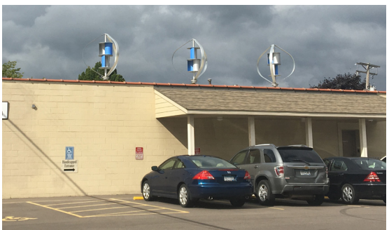
Existing wind energy conversion systems in place at Capitol Lien, 1010 Dale St N.
