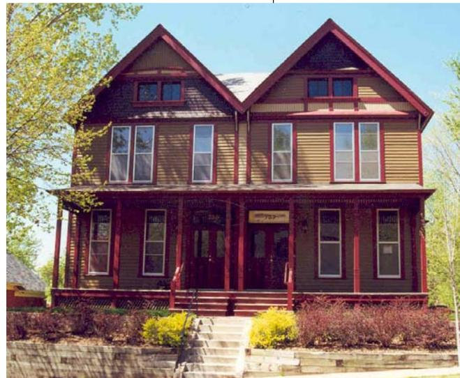
*735-737 E. 5th Street, before photo at left, after photo above showing reconstructed front porch, restored siding and an appropriate paint scheme.*
