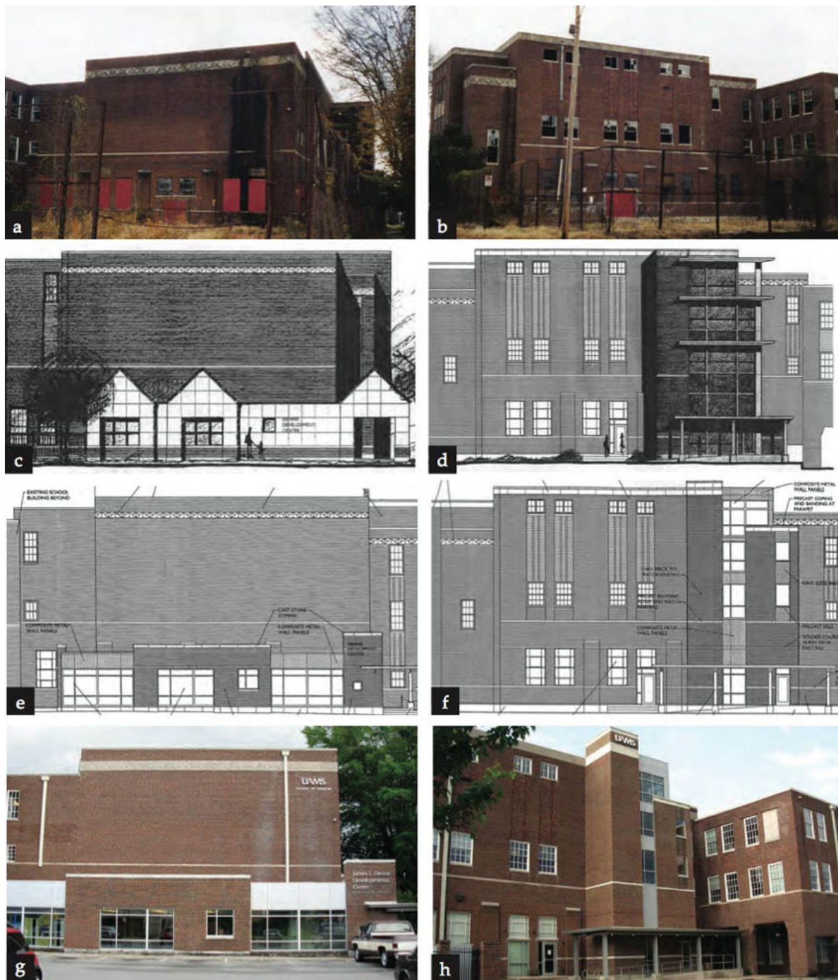
Figure 15 (above). The rehabilitation of a c. 1930 high school auditorium for a clinic and offices proposed two additions: a one-story entrance and reception area on this elevation (a); and a four-story elevator and stair tower on another side (b). The gabled entrance (c) first proposed was not compatible with the flat-roofed auditorium and the design of the proposed stair tower (d) was also incompatible and overwhelmed the historic building. The designs were revised (e-f) resulting in new additions that meet the Standards (g-h).
