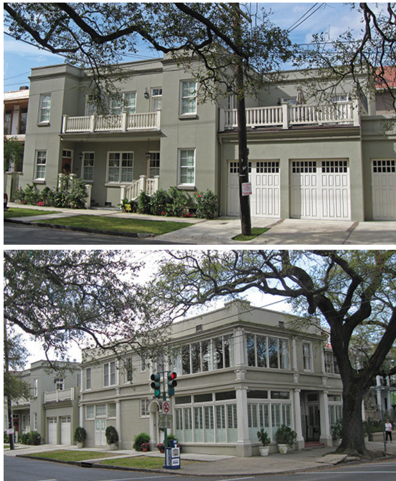
Figure 5. This addition (top left) is constructed of matching brick and attached by a recessed connector (top right) to the 1914 apartment building (bottom left). The design is compatible and the addition is smaller and subordinate to the historic building (bottom right).
