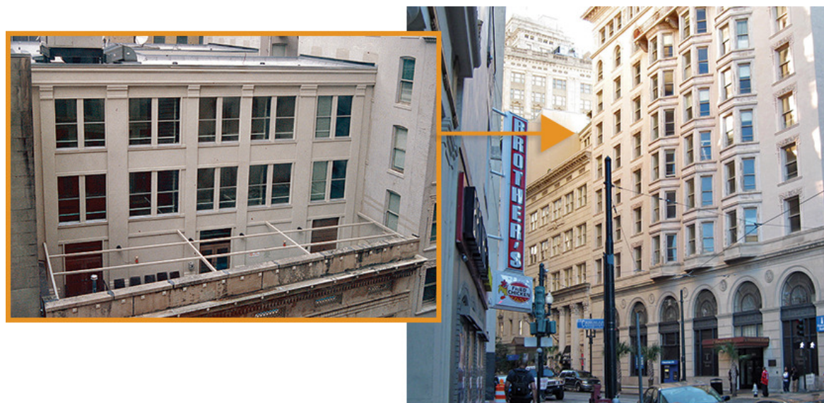
Figure 25. It was possible to add a compatible, three-story, penthouse addition to the roof of this five-story, historic bank building because the addition is set far back, it is surrounded by taller buildings and a deep parapet conceals almost all of the addition from below.
