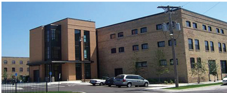
Figure 8. The rehabilitation of this large, early-20th century warehouse (top) into affordable artists’ lofts included the addition of a compatible glass and brick elevator/stair tower at the back (bottom).
