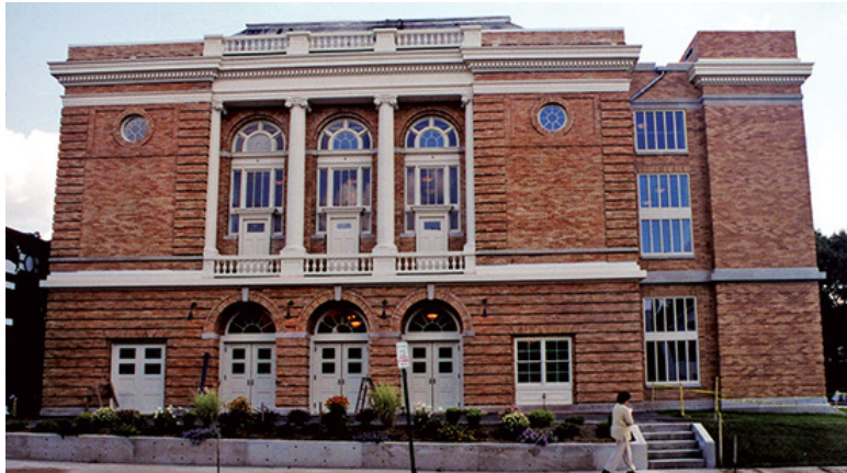
Figure 7. A vacant side lot was the only place a new stair tower could be built when this 1903 theater was rehabilitated as a performing arts center. Constructed with matching materials, the stair tower is set back with a recessed connector and, despite its prominent location, it is clearly subordinate and differentiated from the historic theater.
