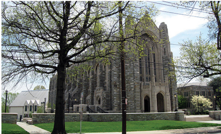
Figure 11. The addition to this early-20th century Gothic Revival-style church provides space for offices, a great hall for gatherings and an accessible entrance (top). The stucco finish, metal roof, narrow gables and the Gothic-arched entrance complement the architecture of the historic church. Placing the addition in back where the ground slopes away ensures that it is subordinate and minimizes its impact on the church (bottom).
