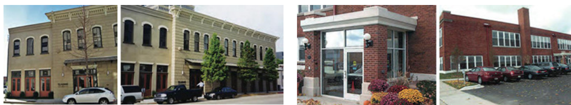
Figure 27b. Although the new brick stair/elevator tower (27a) is not visible from the front (27b), it is on a prominent side elevation of this 1890 stone bank. The compatible addition is set back and does not compete with the historic building. Photos: Chadd Gossmann, Aurora Photography, LLC.
