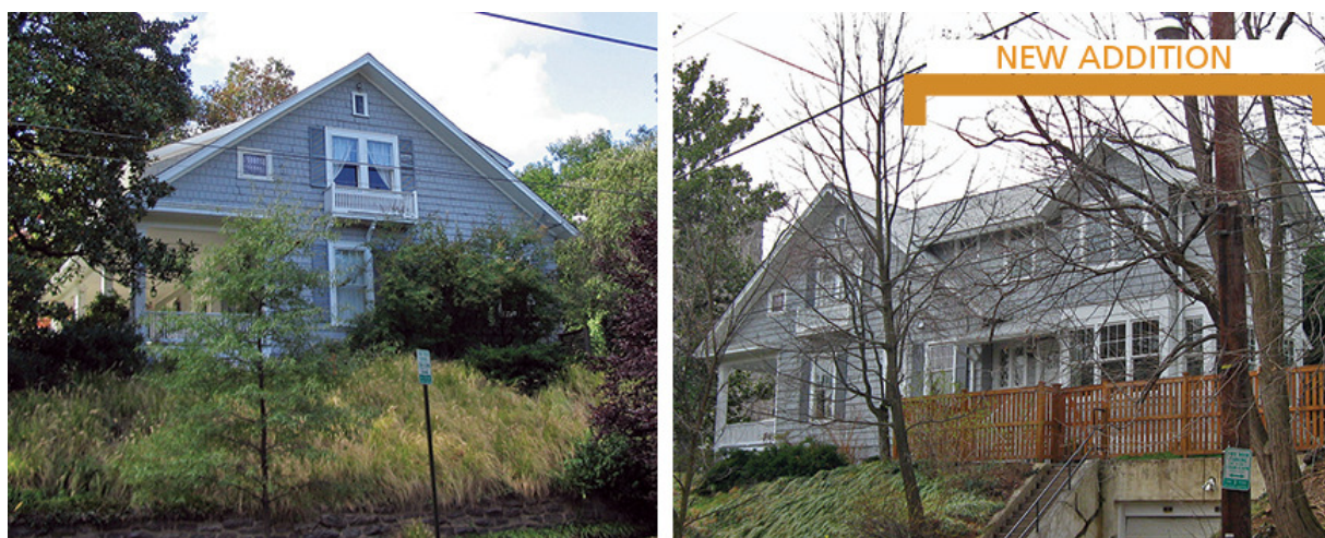
Figure 18. The expansion of a one- and one-half story historic bungalow (left) with a large two-story rear addition (right) has greatly altered and obscured its distinctive shape and form.
