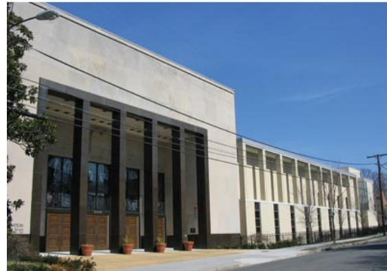
Figure 12. This 1954 synagogue (top) is accessed through a monumental entrance to the right. The new education wing (bottom) added to it features the same vertical elements and color and, even though it is quite large, its smaller scale and height ensure that it is secondary to the historic resource.
