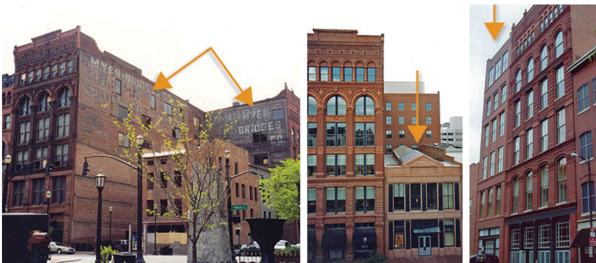
Figure 21. Both wings of this historic L-shaped building (above, left), which fronts on two city streets, adjoined vacant lots. A two-story addition was constructed on one lot (above, middle) and a six-story addition was built on the other (above, right). Like the historic building, which has two different facades, the compatible new additions are also different and appear to be separate structures rather than part of the historic building.
