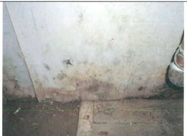
Basement north side—Mold present on the lower and mid portion of the wall as well as water damage to sheetrock.
