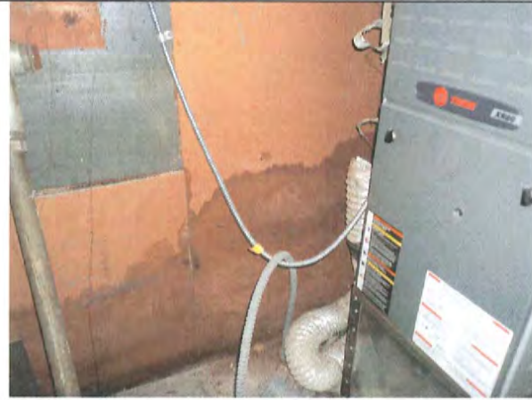
208 First Floor—saturated sheetrock present near furnace in utility room. It was wet at time of visit.
