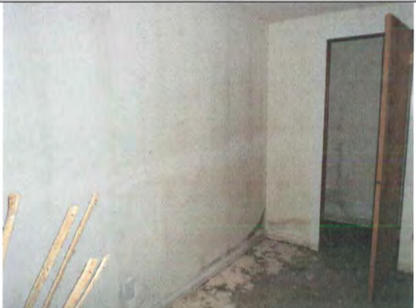
210 First Floor—East room: mold on walls. Note evidence on walls of wet studs. Floor was wet at time of visit.
