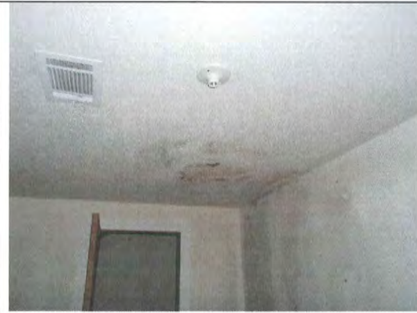
208 First Floor—east room: ceiling and wall mold.
