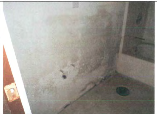
208 First Floor—mold present along bathroom walls.
