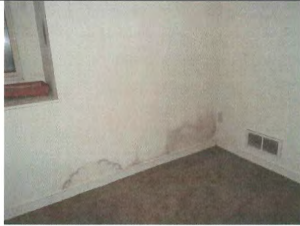
210 First Floor—mold present on the lower portion of the wall NE-central room.
