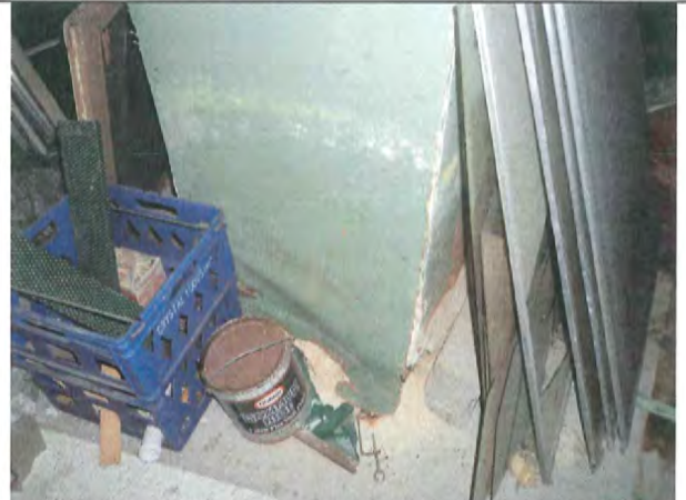
Basement south side—SW area: water damage to sheetrock.
