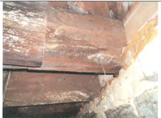
Basement central corridor—mold present on floor joist.
