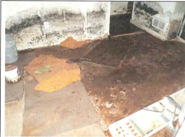
208 First Floor—kitchen: standing water on floors and saturated carpet plus mold were present on the kitchen floor and walls.
