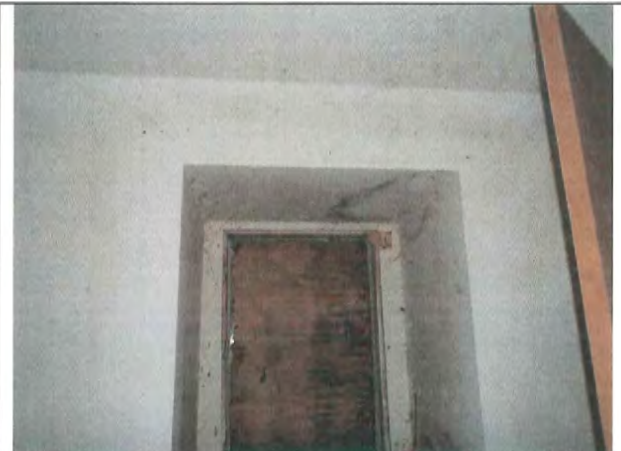
208 First Floor—east room: mold around window area.
