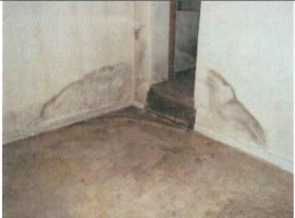
210 First Floor—mold present on the lower and mid portions of the walls in the room off kitchen. Floor was wet at time of visit.
