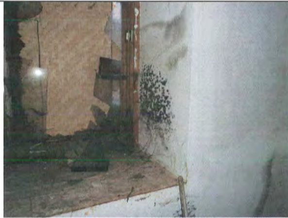
210 First Floor—East room mold present around window.
