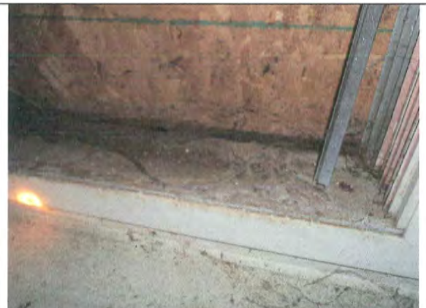
210 First Floor—NW-central room window well: mold
