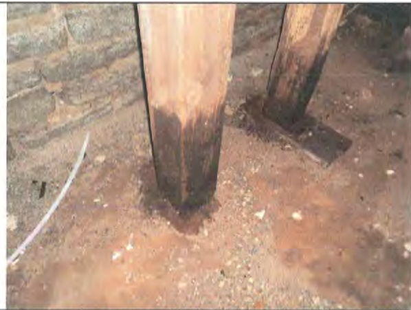
Basement central corridor—water saturated on support beams
