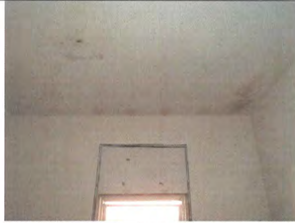
210 2 nd Floor—NE-central room. Staining and mold present on ceiling.
