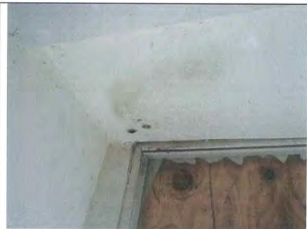
208 First Floor—SE-central room: mold present adjacent to window.
