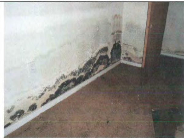
208 First Floor—mold present along lower portion of walls, east room. Floor and wall base were wet at time of visit.
