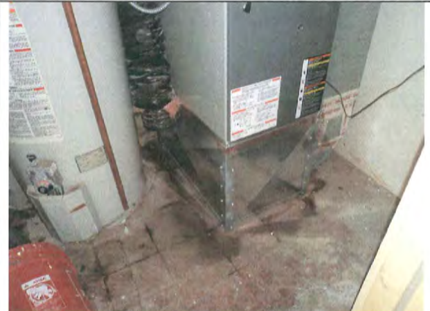
210 First Floor—floor in utility room wet at time of visit.
