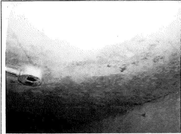
Basement north side—Mold and water damage present on the ceiling sheetrock.
