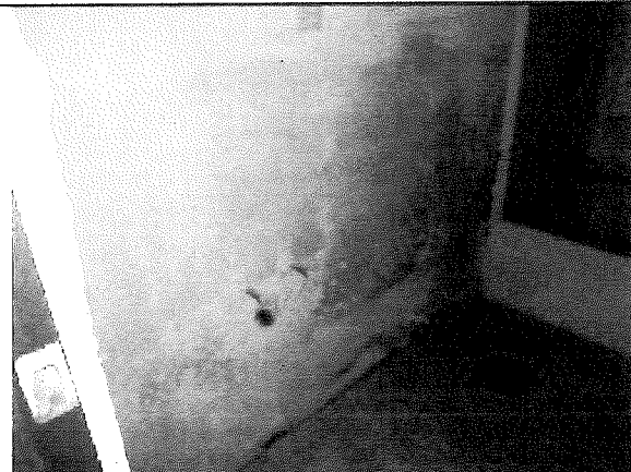
208 First Floor—mold present along bathroom walls.
