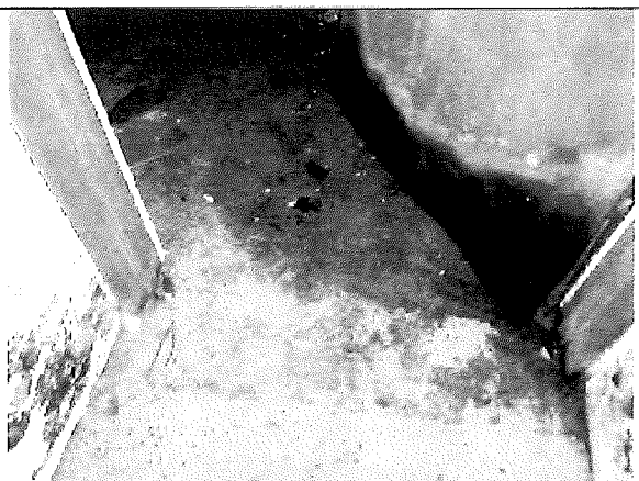
208 First Floor—east room: mold present on walls, flooring, door and door frame. Water present in building materials.
