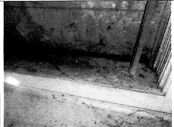
210 First Floor—NW-central room window well: mold
