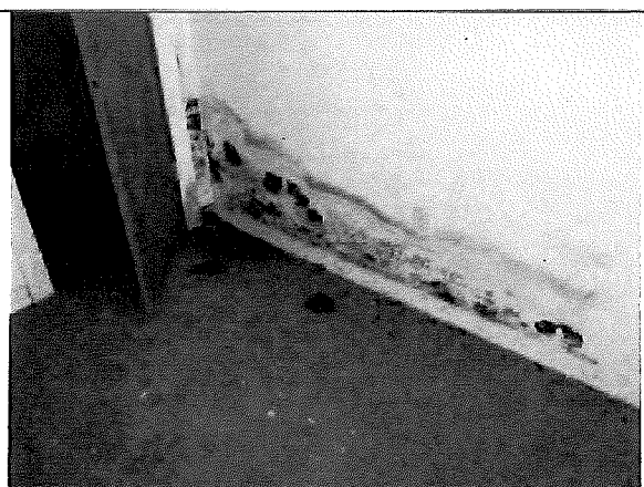
208 First Floor—SE-central room: saturated carpet and wet floors were present with mold located on the lower portion of the walls.
