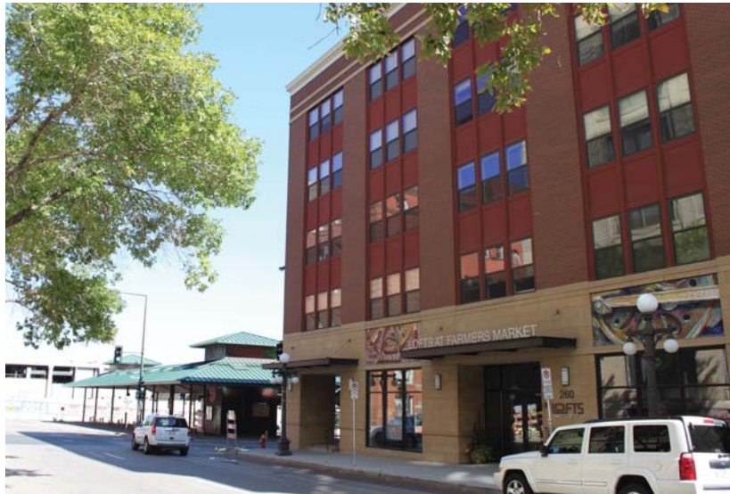
The Lofts at Farmers Market in Saint Paul's Lowertown neighborhood is an example of a new construction project that has complied with the Sustainable Building Policy.
