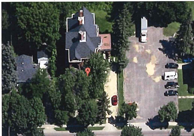
Aerial showing driveway width and parking availability
