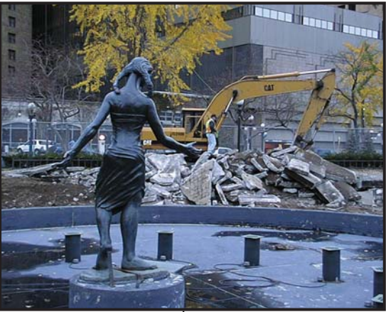
2000 Steps removed for ADA accessibility. Fountain rebuilt, pumps replaced, electrical service upgrade to provide for increased capacity. New circular plaza benches path benches and concrete planters added.
