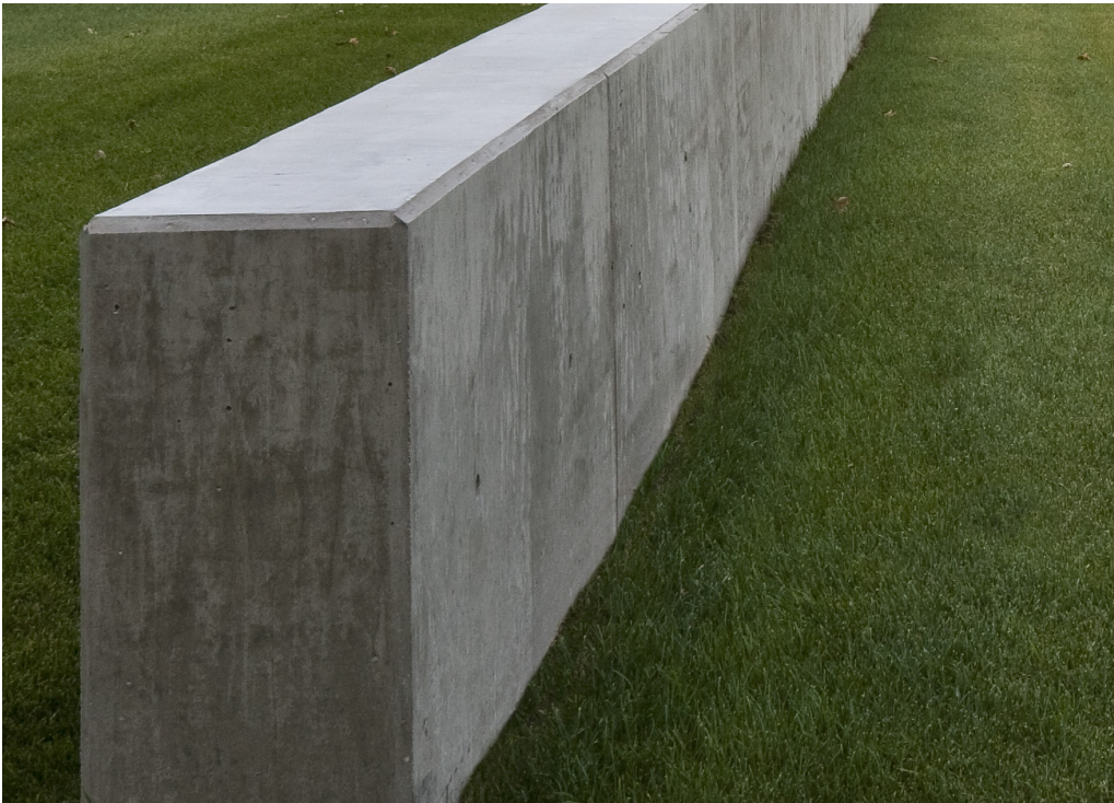
edges and top: 1/2" chamfer
