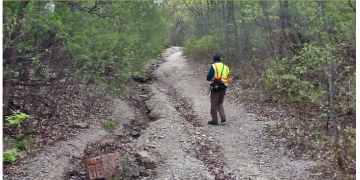
Photo: Erosion on the Brickyard Trail–Fossil/Brick Oven Section. Moderate-to-severe erosion from concentrated stormwater runoff along the straight and steep sections of the Brickyard Trail was observed. A steep slope adjacent to the trail showed evidence of slope failure that was reactivated during a wet period in June 2014.
