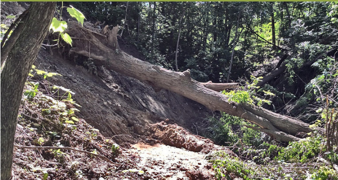
Photo: Ravine slope failure. Significant erosion was observed along the ravine side slopes; there are several active slope failures in the ravine.
