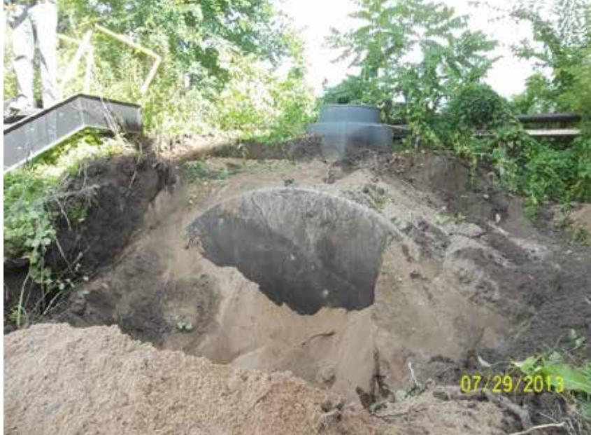
A photograph showing the early stages of soil excavation around an underground storage tank (UST). A large, dark, cylindrical object is partially buried in the earth. The ground is uneven and appears to be disturbed. In the background, there are trees and some industrial structures, including a green tank and a building with a yellow frame. A date stamp "07/29/2013" is visible in the bottom right corner of the photo. |
