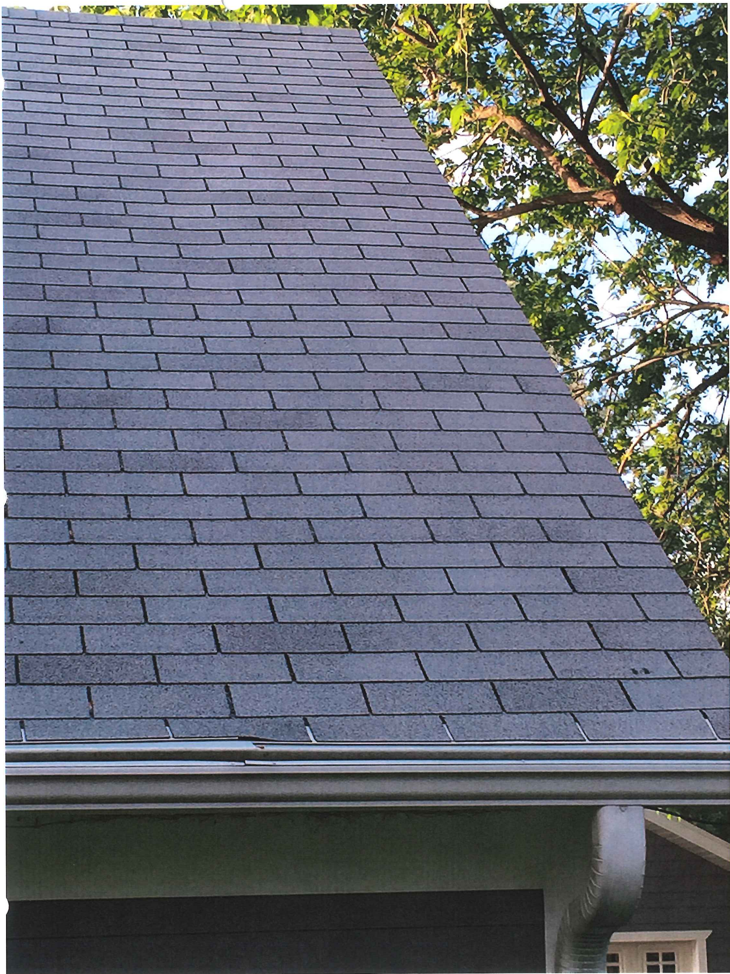
1373 Summit Ave - Existing Asphalt Roof
