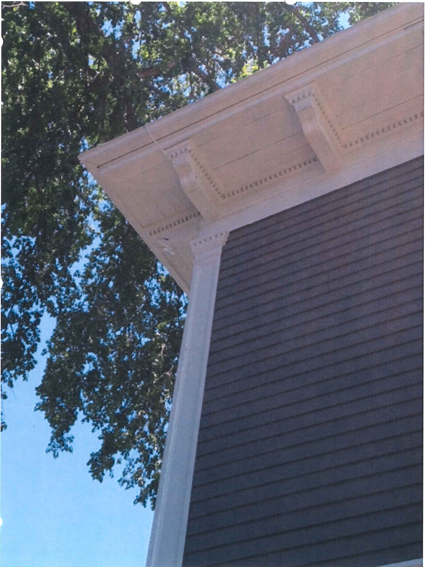
1373 Summit Ave - Typical Soffit-Bracket-Corner Detail
