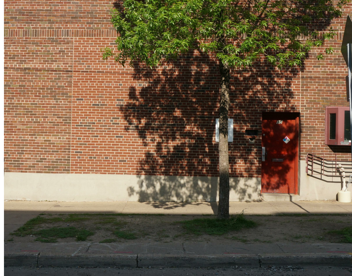
3 BRICKED-IN OPENING W/ MAN DOOR
