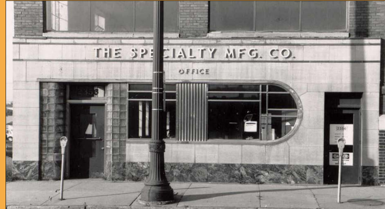
FIGURE 1.3 - Detail of the Specialty Manufacturing Company, built 1906.
