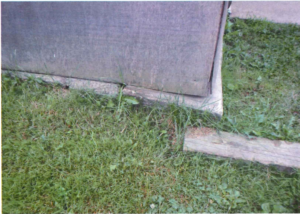
Photo 9- Signs of movement in concrete supporting stud walls of one story shed on west side of building
