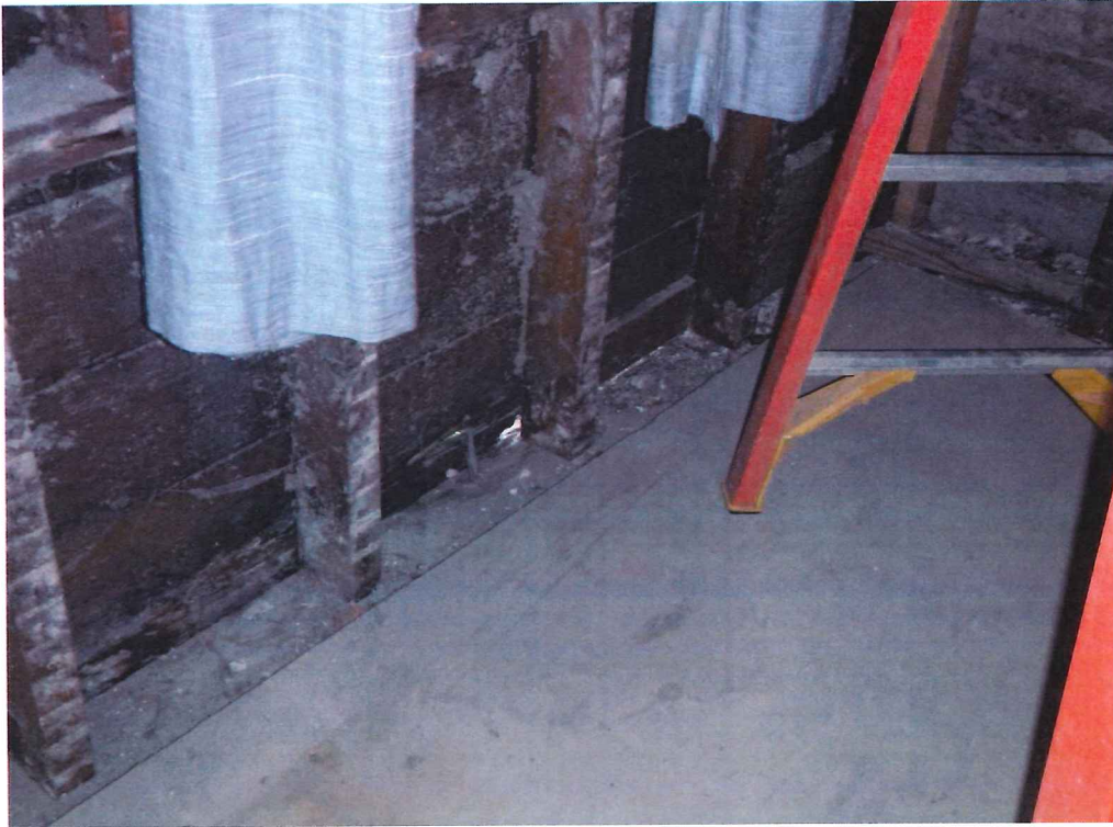
Photo 3- Openings in exterior stud wall
