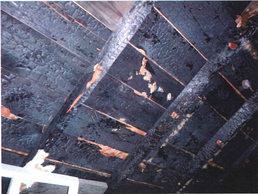
Photo 1- Fire damage at roof level
