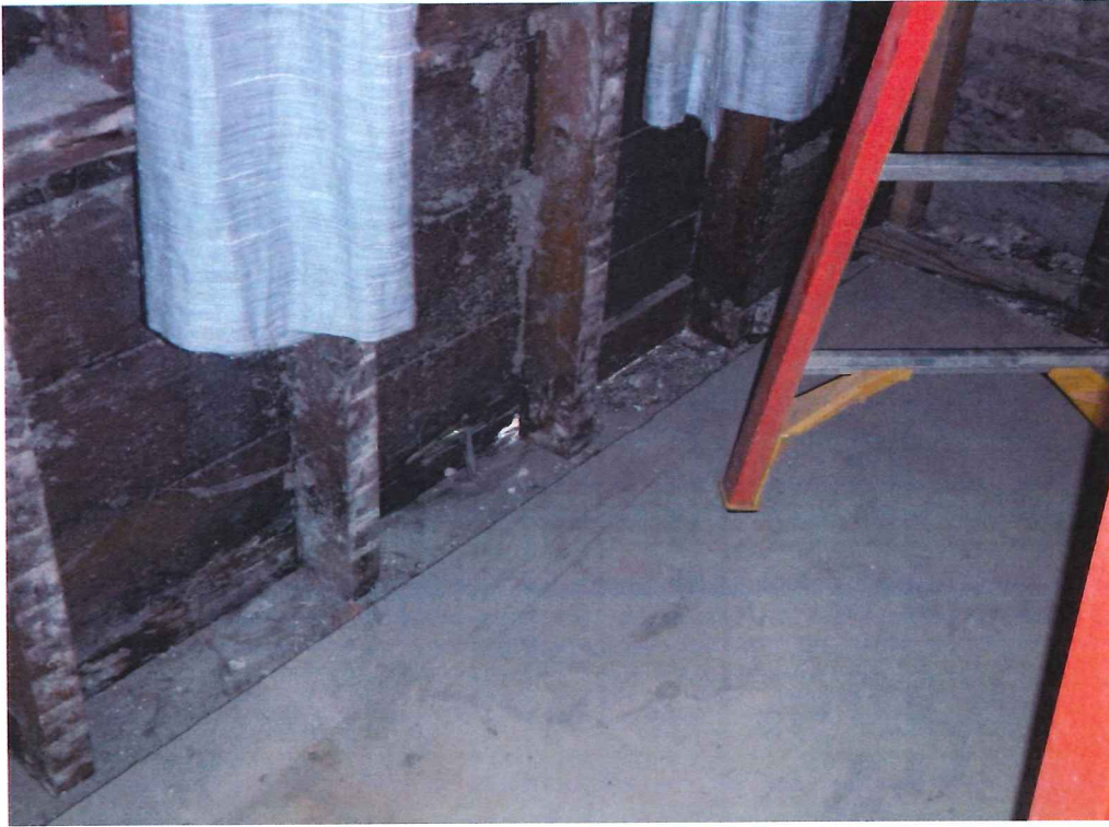
Photo 3- Openings in exterior stud wall
