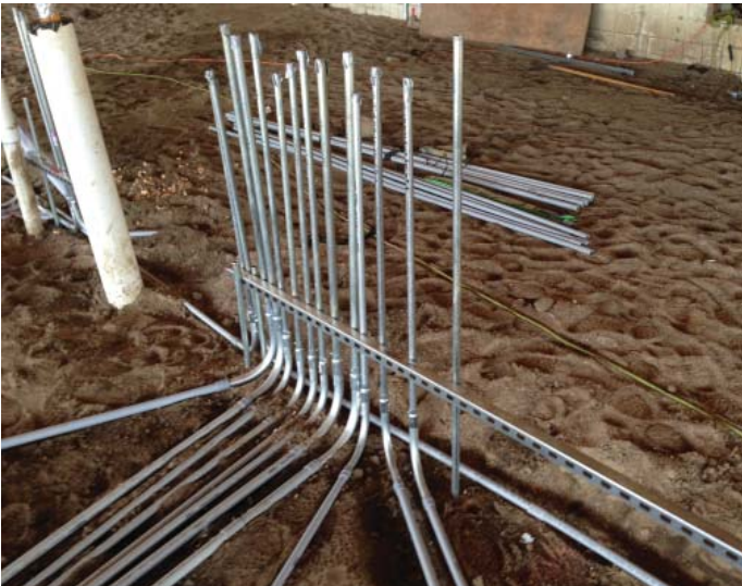
5. Placing conduits for installation in future walls (8/26/15)
