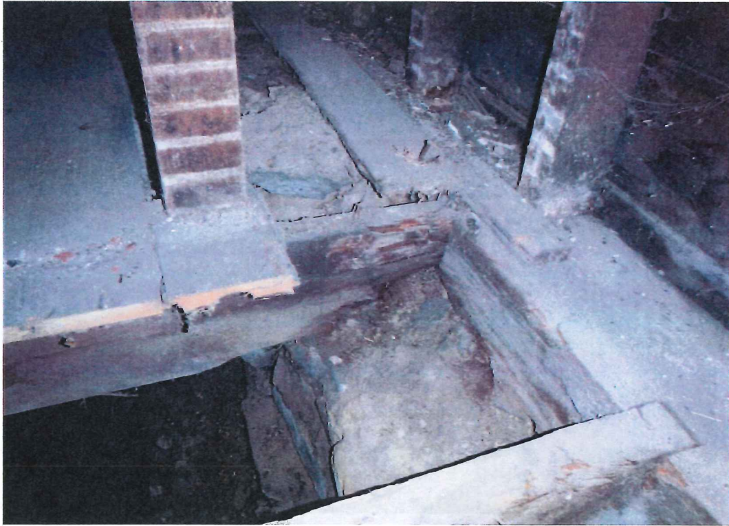
Photo 7- Deteriorated joists and sill at bearing on stone foundation wall
