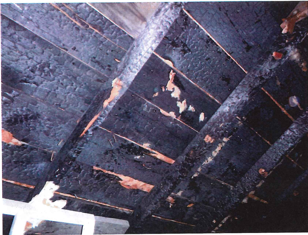
Photo 1- Fire damage at roof level
