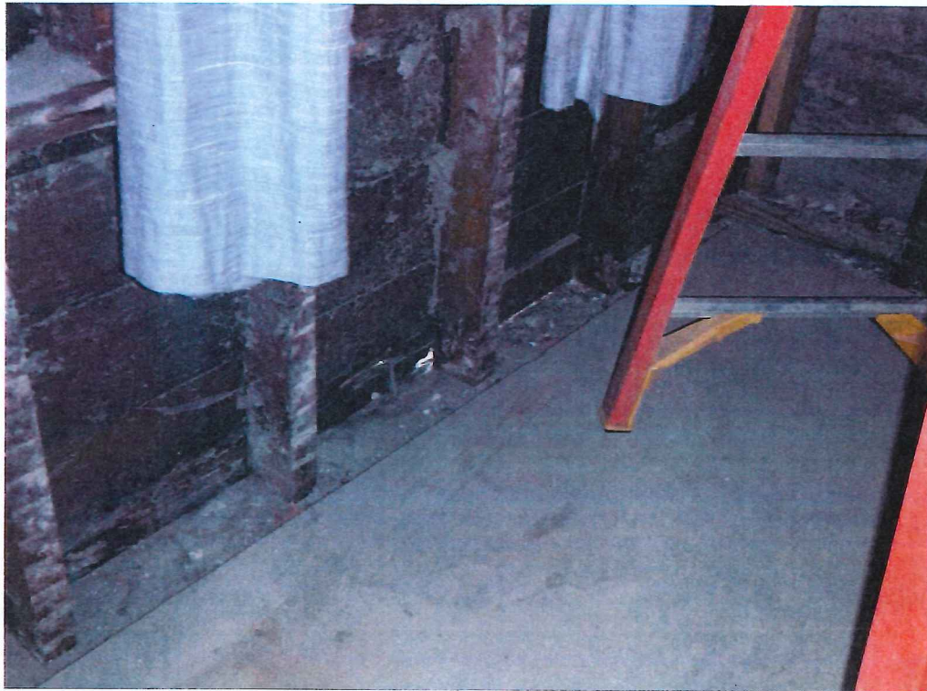
Photo 3- Openings in exterior stud wall
