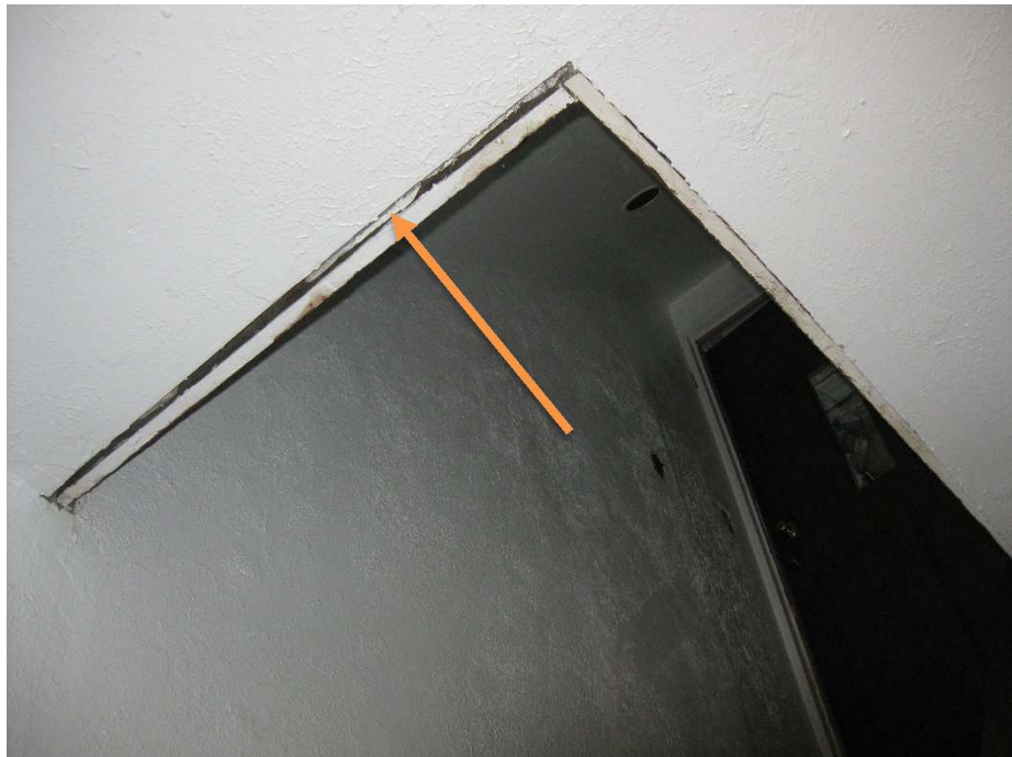
Picture 4 – Gap Due to Sloping
