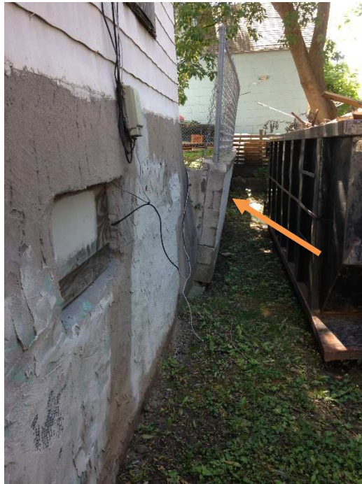
Picture 10 – Retaining Wall Out of Plumb
