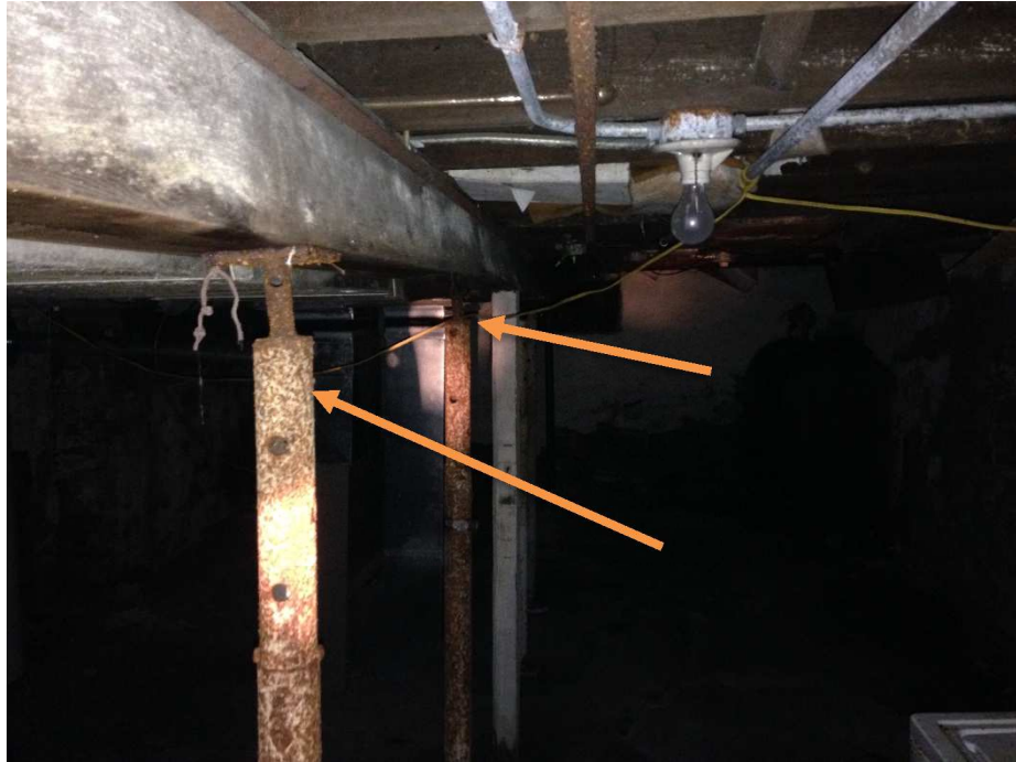
Picture 9 – Shoring Columns Supporting a Beam
