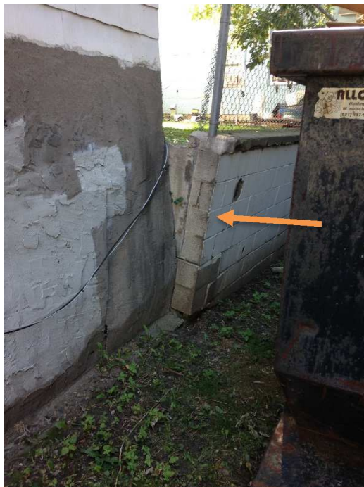
Picture 11 – Retaining Wall Out of Plumb
