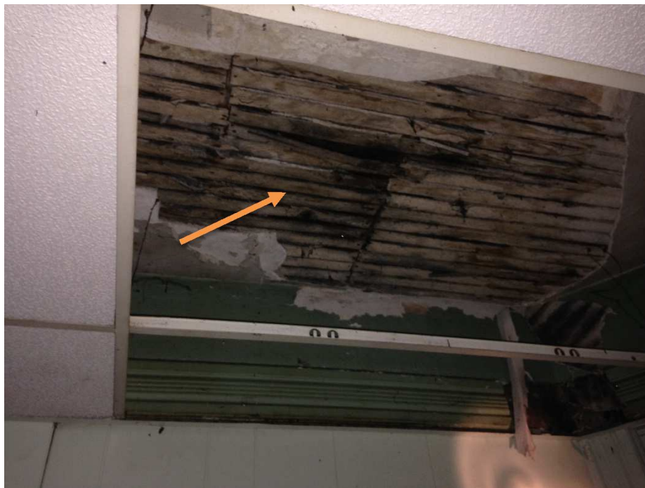
Picture 6 – Deterioration of Ceiling System
