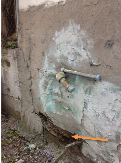
Picture 12 – Stucco Deterioration
