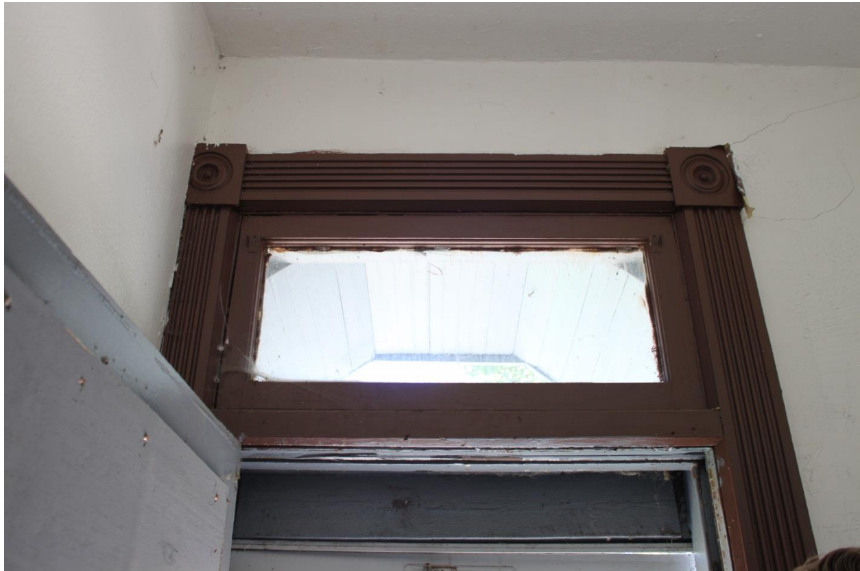
Transom and trim detail of front door in first floor vestibule (above), similar trim detail in upstairs front room (below)
