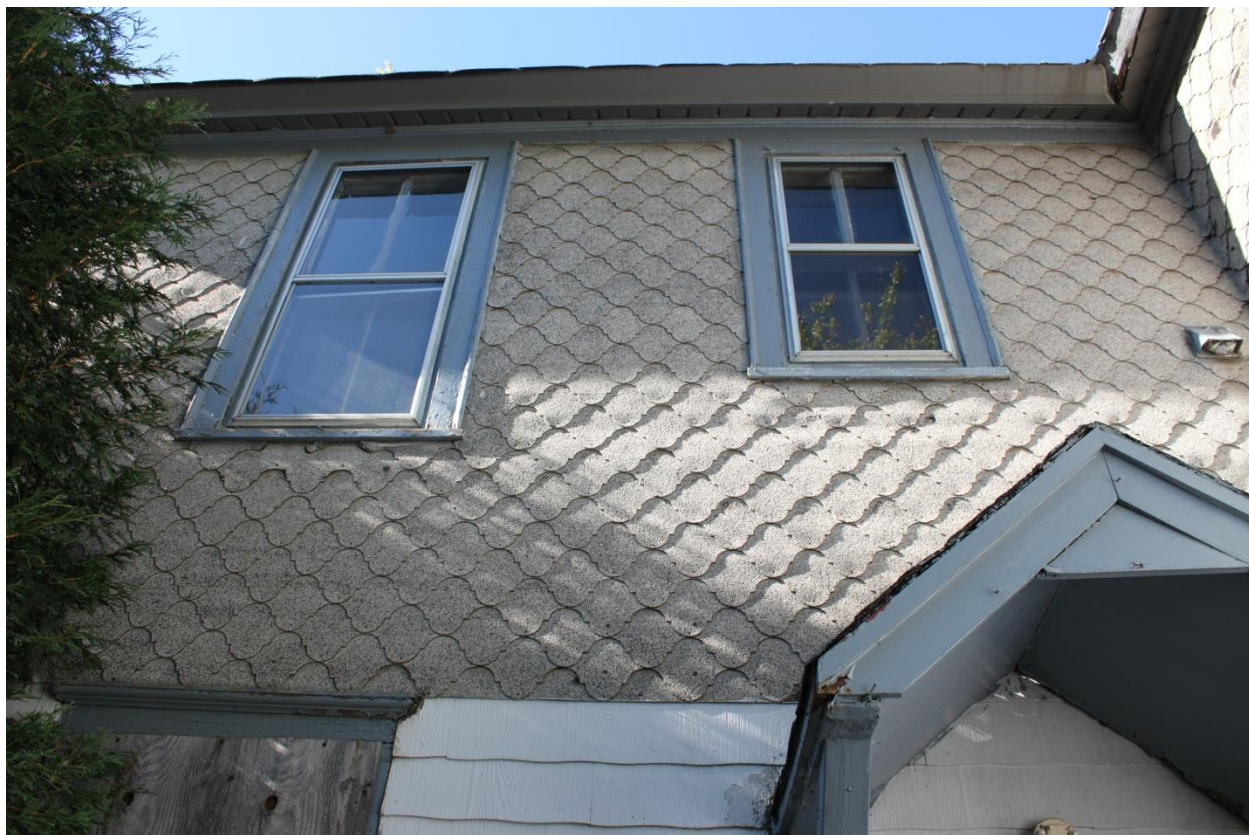
C. 1935 asphalt and asbestos cement shingle detail on north elevation (above), c. 1884 Eastlake style balusters and newel post detail in front hallway (below)
