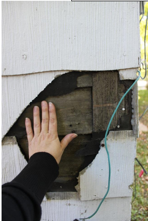
275 Bates Avenue southeast elevation (top), c. 1935 asbestos cement and asphalt shingle exterior walls (below) with exposed original clapboard (below left)
