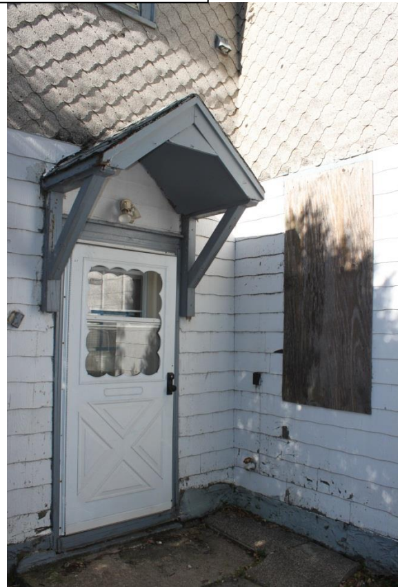
275 Bates Avenue southeast elevation (top), c. 1935 asbestos cement and asphalt shingle exterior walls (below) with exposed original clapboard (below left)
