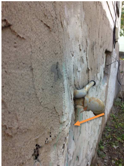
Picture 13 – Stucco Bulging Out
