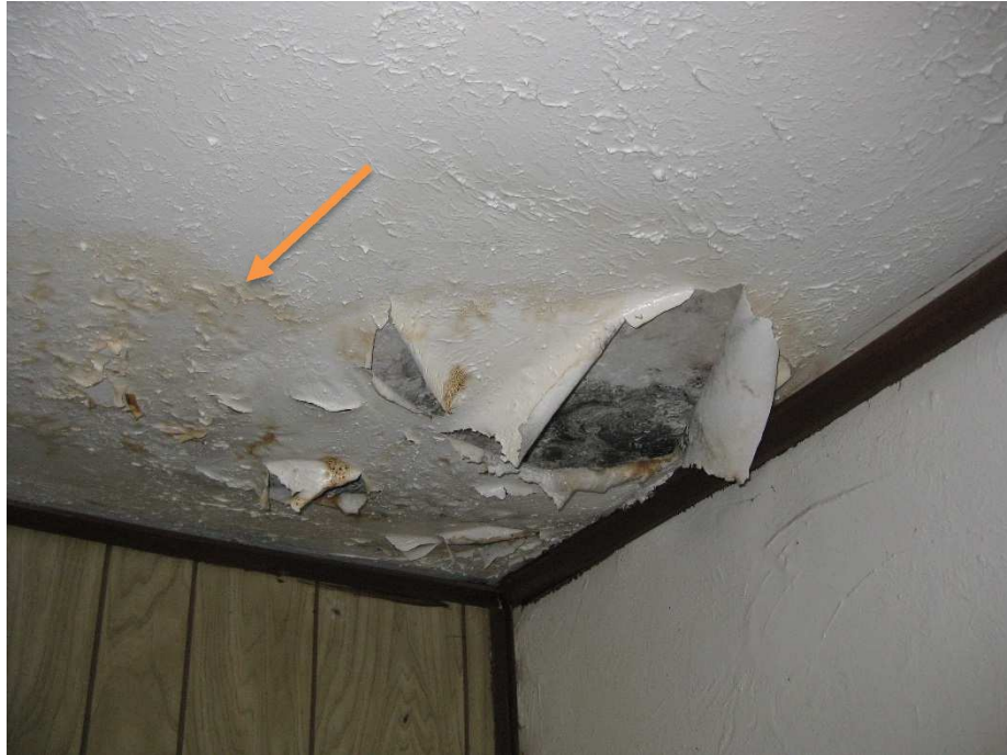
Picture 5 – Water Damage on Second Floor Ceiling
