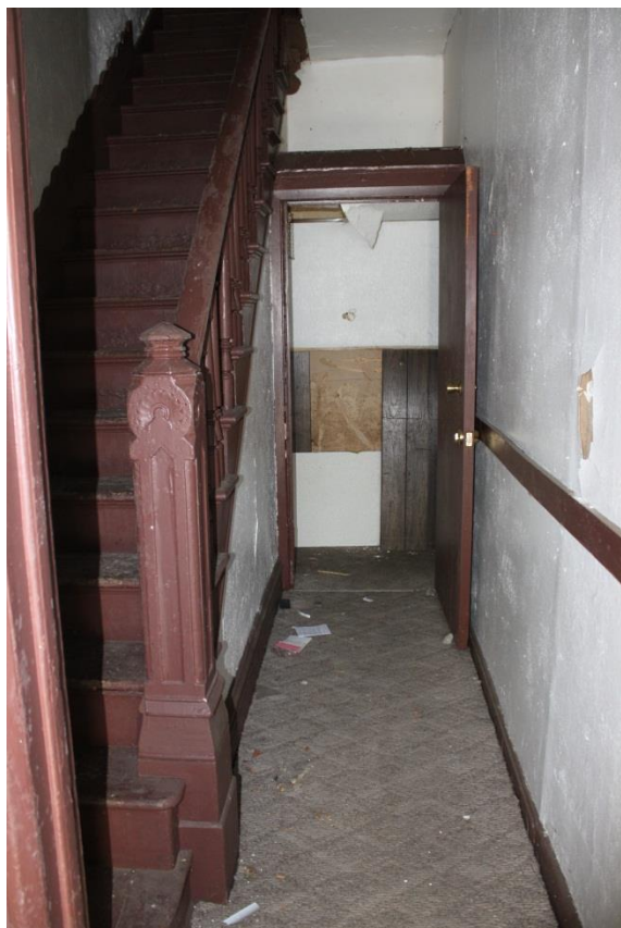
C. 1935 asphalt and asbestos cement shingle detail on north elevation (above), c. 1884 Eastlake style balusters and newel post detail in front hallway (below)
