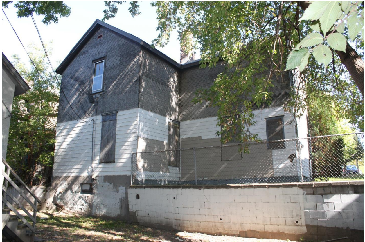
275 Bates Avenue southeast elevation (top), c. 1935 asbestos cement and asphalt shingle exterior walls (below) with exposed original clapboard (below left)
