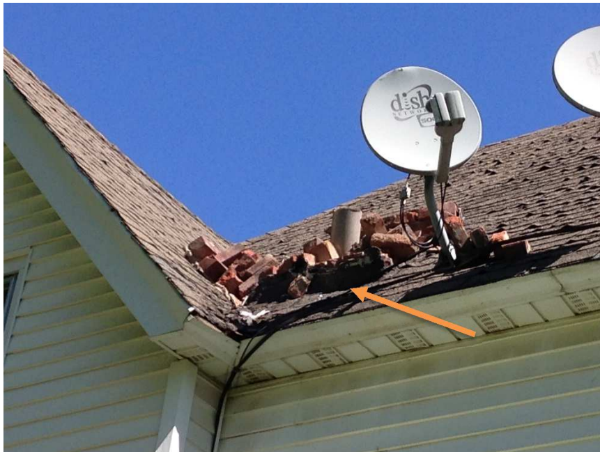
Picture 7 – Demolished Chimney
