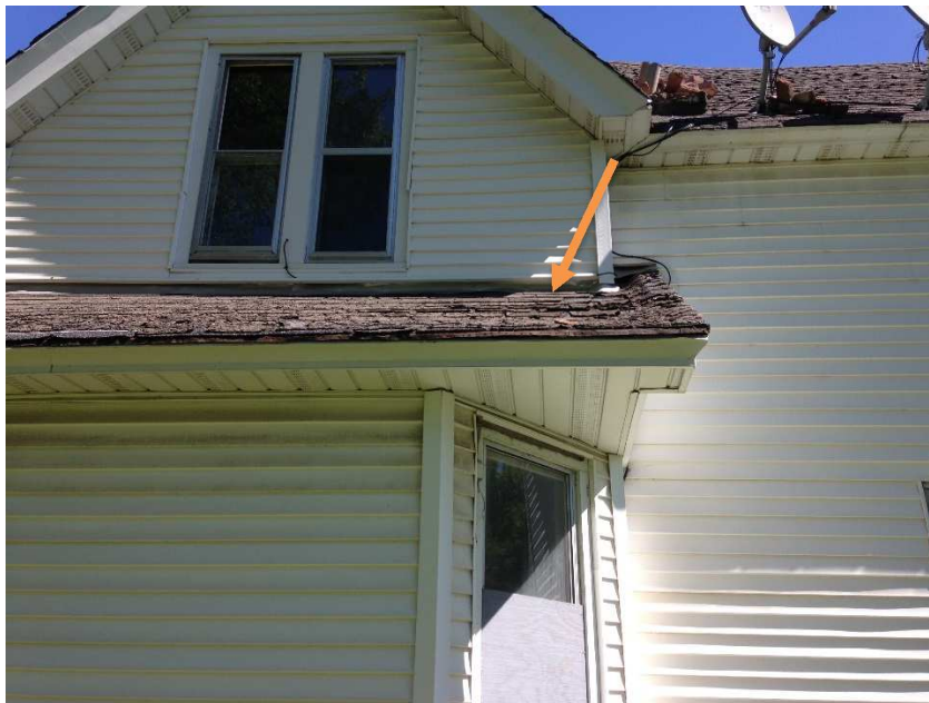
Picture 9 – Roof Sag on the West Side
