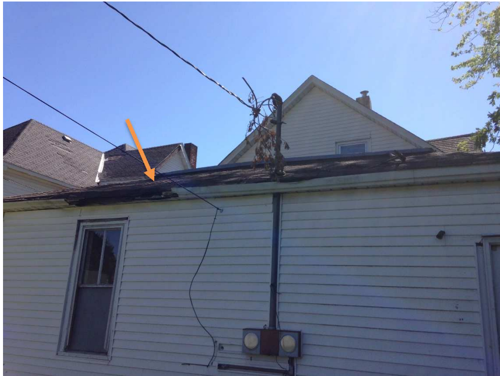
Picture 10 – Rot At Back Roof
