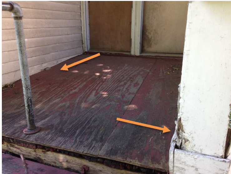
Picture 5 – Front Porch Deterioration and Slope
