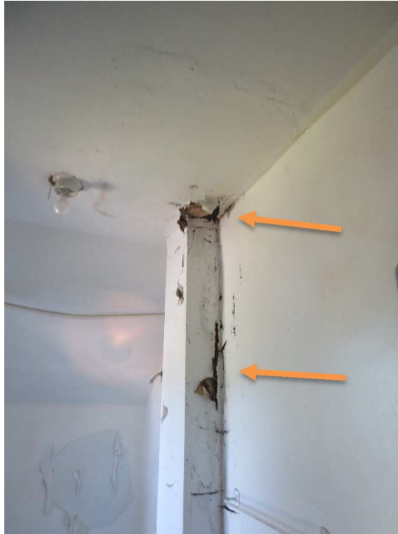
Picture 16 – Water Damage to Column
