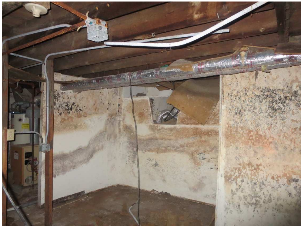
Picture 18 – Mold in Basement
