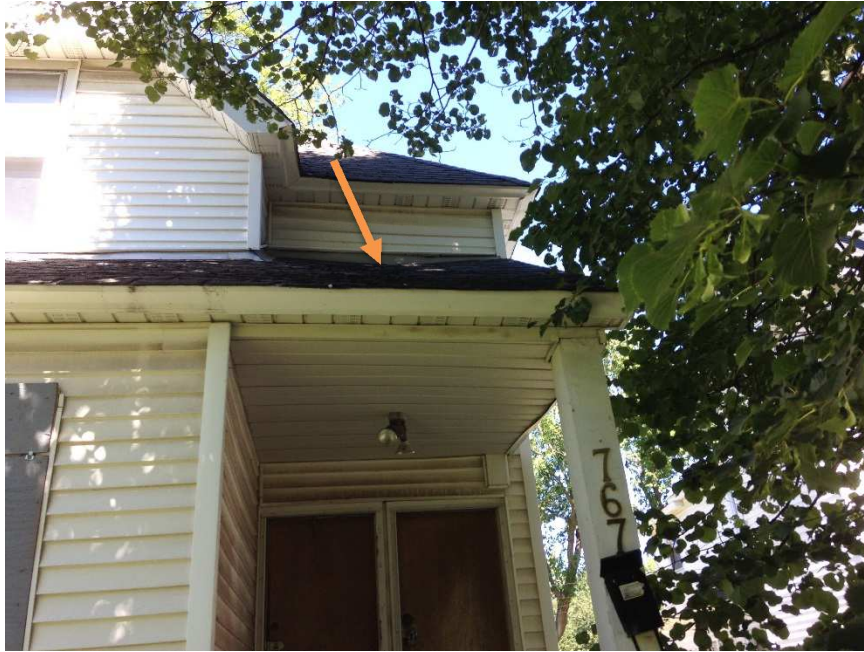
Picture 8 – Roof Sag at the Front Porch
