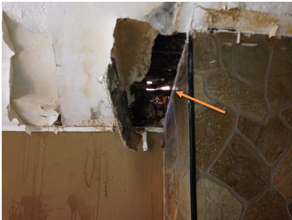
Picture 11 – Rot Through Roof
