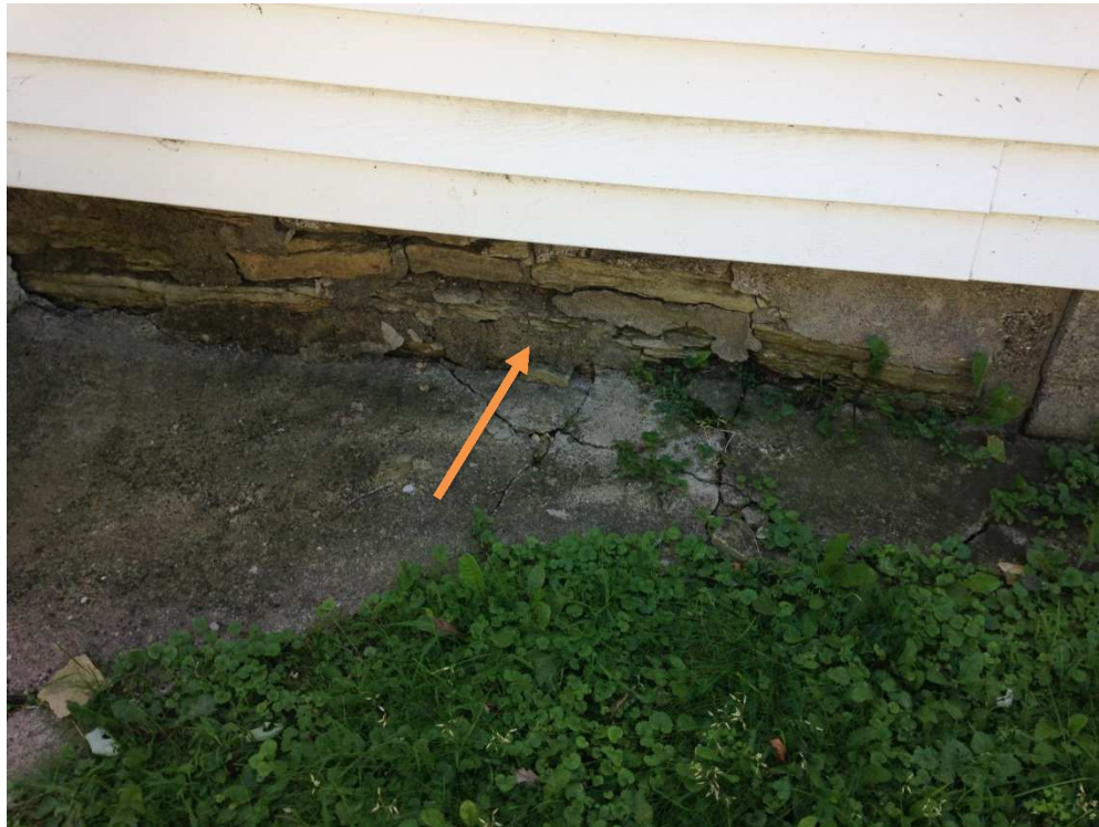
Picture 12 – Foundation Deterioration
