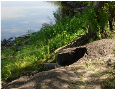
Existing Riverbank Condition
