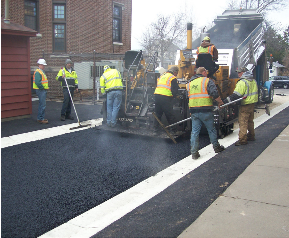
Laying porous asphalt at the Saint Paul's first green alley, Hamline Library, October 2012. Courtesy Wes Saunders-Pearce.
