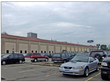
Window openings on the north facade of the main assembly building have been enclosed with concrete block.
