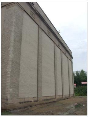
The window openings on the west facade of the steam plant were enclosed following flooding in the 1950s.
