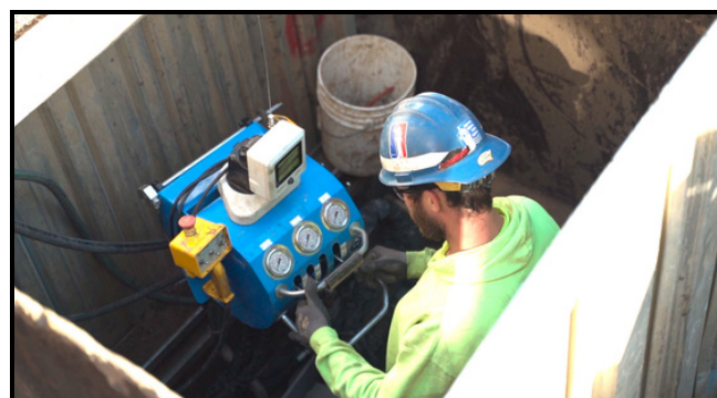
A worker holds copper pipe in a home while another worker guides horizontal drilling equipment underground to allow for a new copper service line to be pulled through from the house to the street during a lead replacement.
