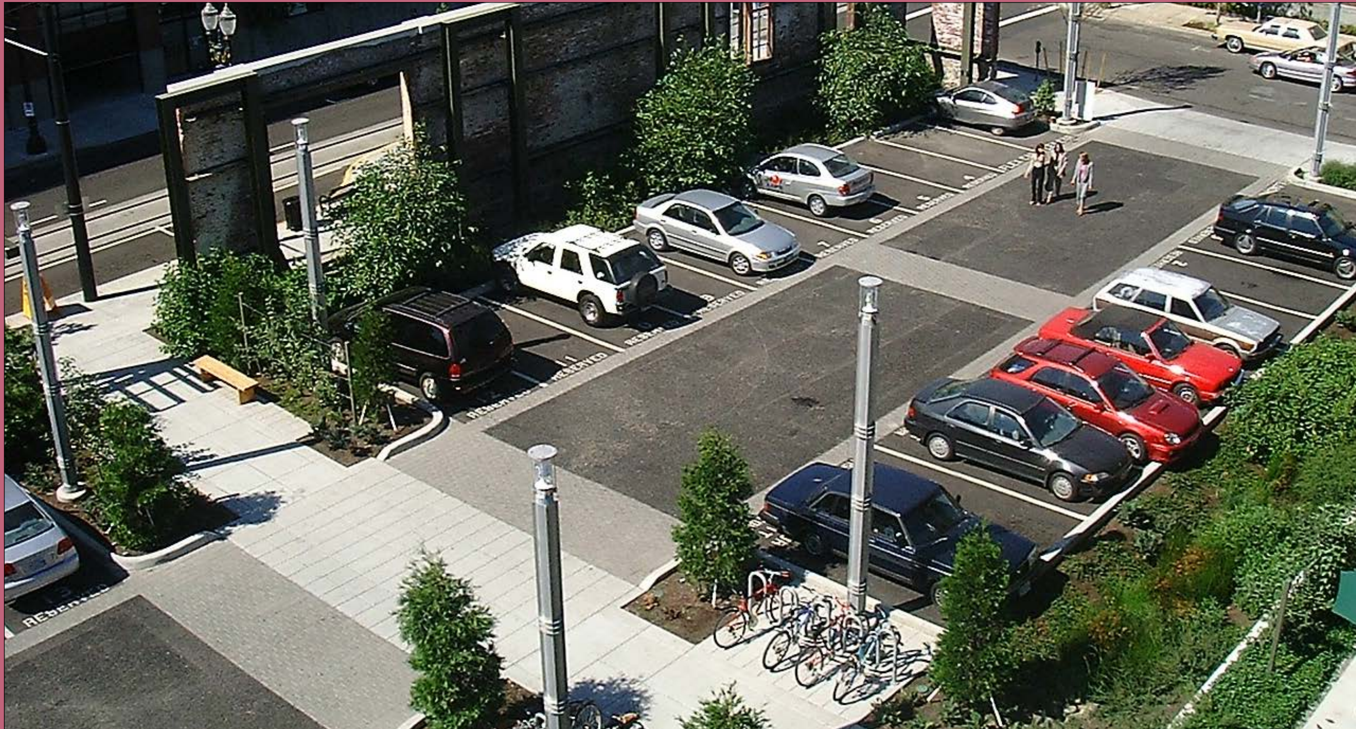
FIGURE 4.9 - A 56-foot wide surface parking lot in Portland, Oregon incorporates features such as permeable paving, integrated bike parking and pedestrian-scaled lighting. It is heavily landscaped and concealed from the street by an integrated former building facade.
