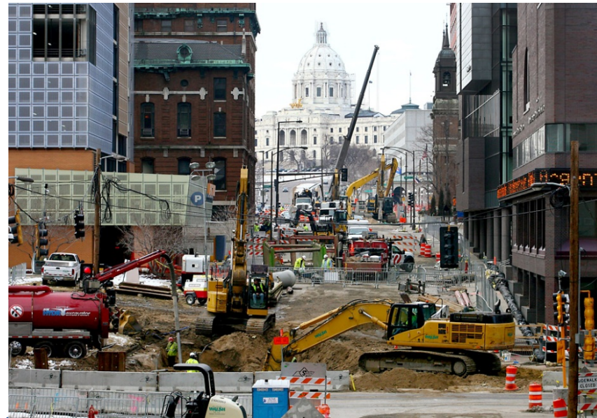
Green Line construction, St. Paul
