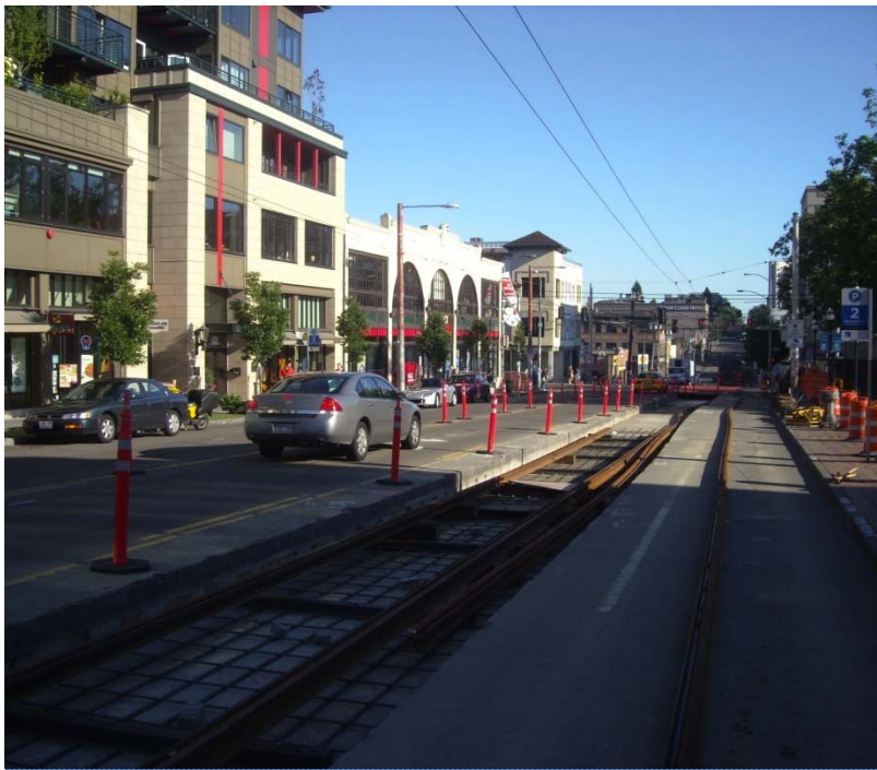
First Hill Streetcar construction, Seattle
