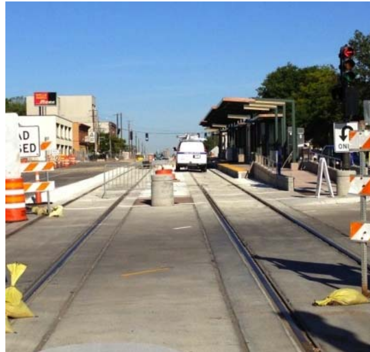
Green Line Construction, St. Paul
