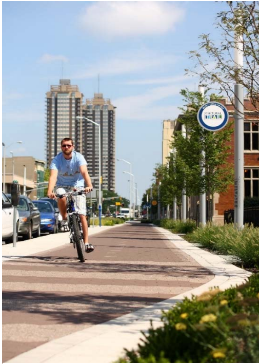
Figure 2 - Raised Protected 2-Way Bike Lane: Indianapolis Cultural Trail (Source: Toole Design Group)
