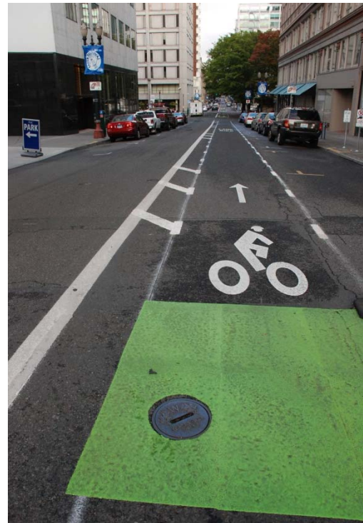
Figure 3 - Buffered Bike Lane (Source: Toole Design Group)
