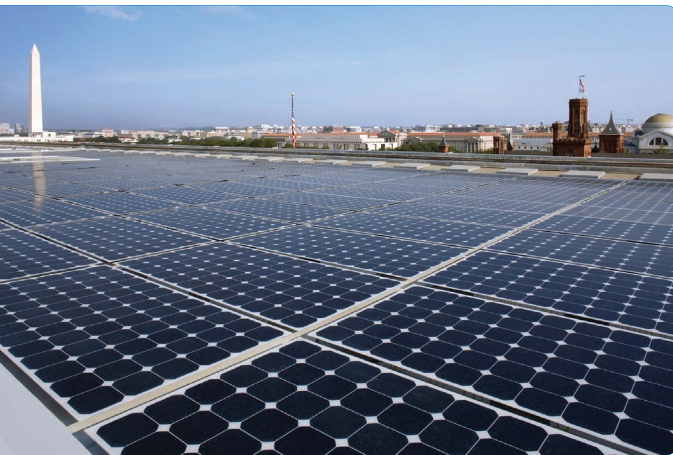
205 kW photovoltaic system installed on the U.S. Department of Energy Forrestal Building in Washington, D.C. (Photo credit: SunPower Corporation)
