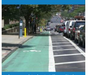
A one-way cycle track protected by a parking lane and buffer and showing optional green paint
