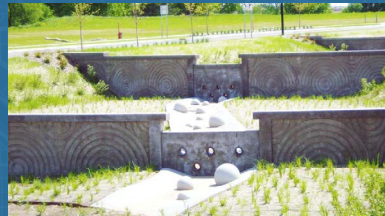
Biofiltration Basin, Tartan Crossing Development City of Oakdale, MN & Wellington Management, Inc.
