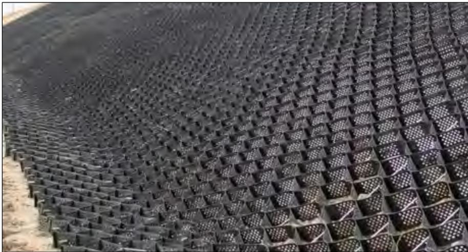
**Photo A-4** Example of geoweb on a steep slope, prior to infill (source: [www.prestogeo.com](http://www.prestogeo.com), used with permission)
