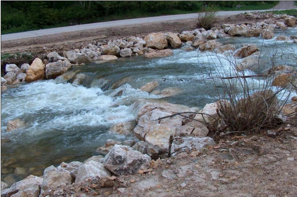
**Photo A-9** Example of a boulder riffle
