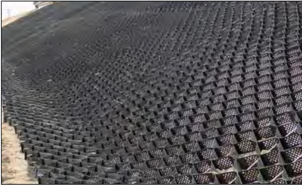
Photo 5-6 Example of Geoweb on a steep slope (prior to infill) (Source: [www.prestogeo.com](http://www.prestogeo.com), used with permission)
