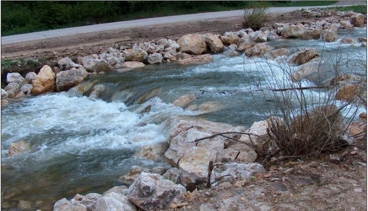
**Photo 5-2**      **Example of a boulder riffle**
