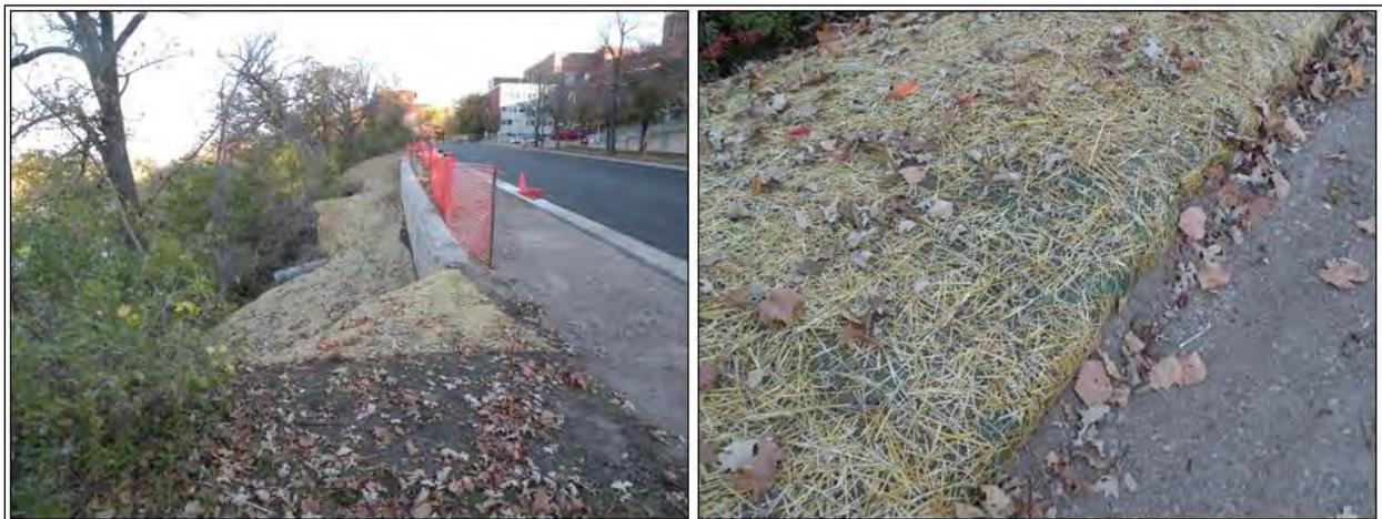
**Photo A-5** Example of a turf-reinforcement mat
