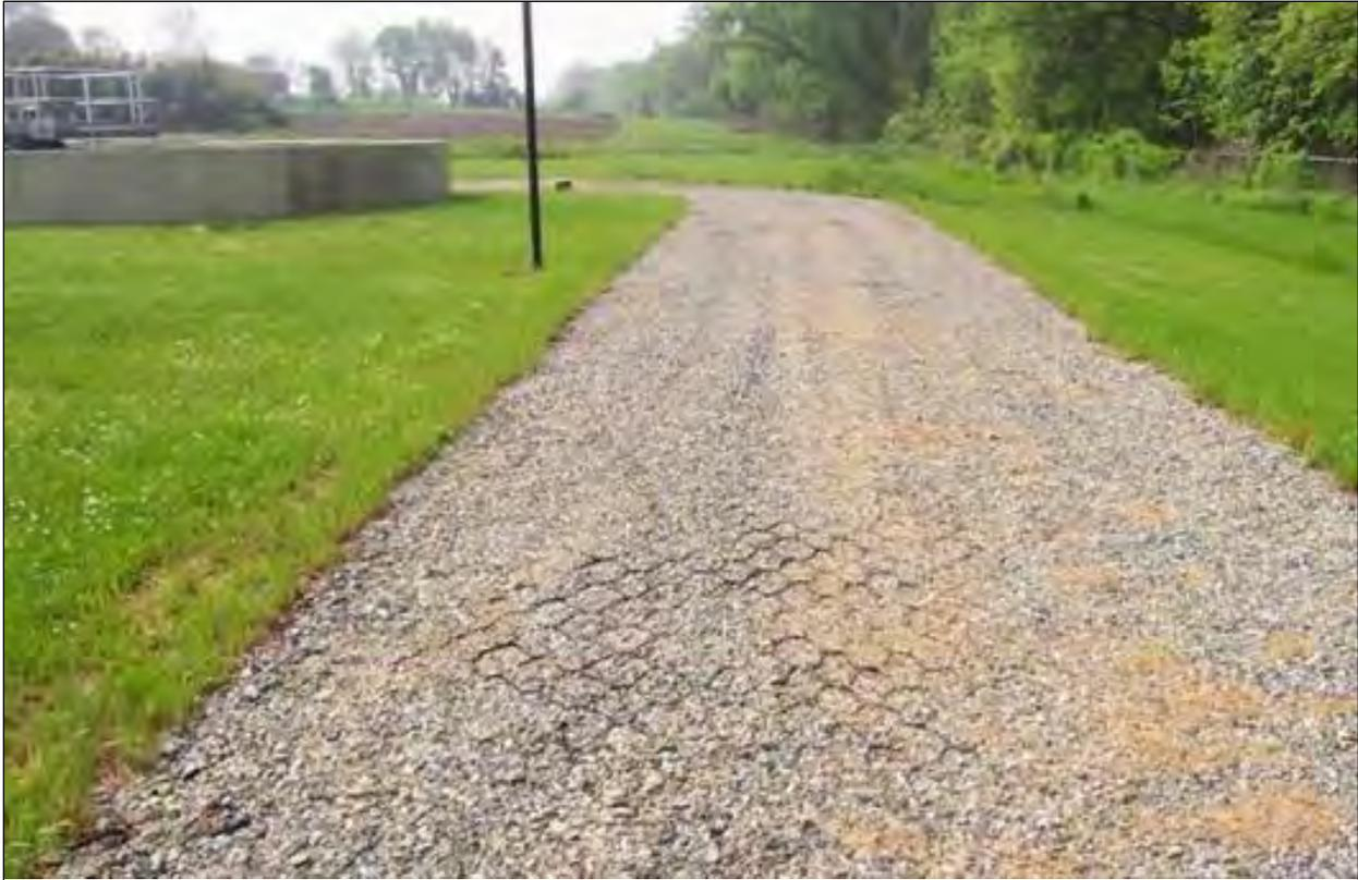
Photo 5-4 Example of Geoweb erosion control (Source: [www.prestogeo.com](http://www.prestogeo.com), used with permission)
