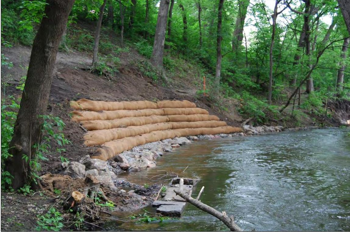
**Photo A-6** Example of vegetated reinforced soil slope (VRSS) before vegetation re-establishes
