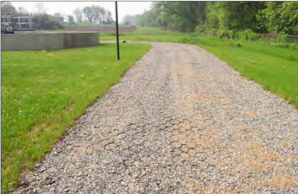
**Photo A-2** Example of geoweb erosion control (source: [www.prestogeo.com](http://www.prestogeo.com), used with permission)
