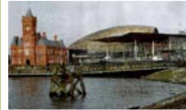
Balance of historic and contemporary roof line treatments.
