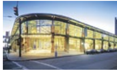
Multiple openings entry points.
