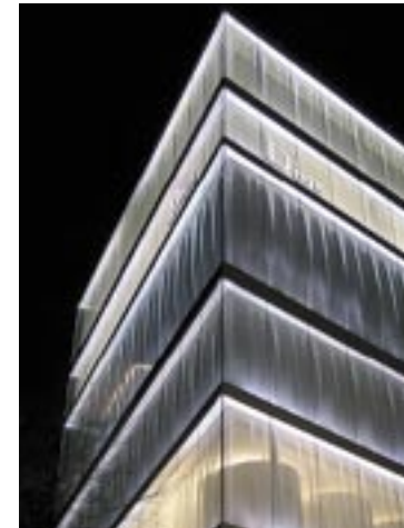
Glass curtain wall creates night quality.
