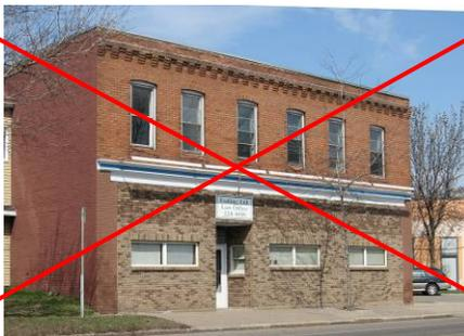
Original first floor windows were removed and the openings were bricked up in the building to the left. The windows installed do not conform with the building's historic character. The narrow rectangular horizontal orientation is incompatible with the age of the structure.
