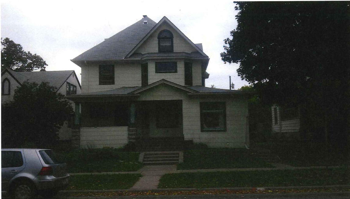
Front of subject property
