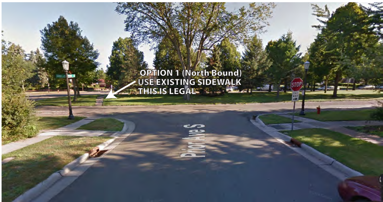
FIG. 1B - VIEW OF EXISTING SIDEWALK
