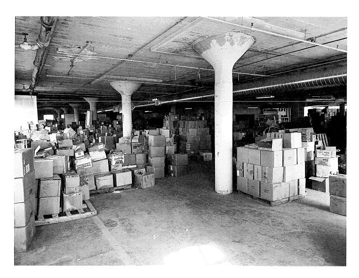
**Photo 12:** St. Paul Casket Company Building, interior view of fourth floor from looking northeast at former production floor, note columns, original sprinkler lines, and yellow workspace demarcation lines.
