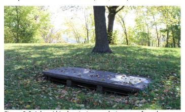
Figure 3.9. Inlet within the picnic area drains water from the perched wetland soils (QEA, 2018).
