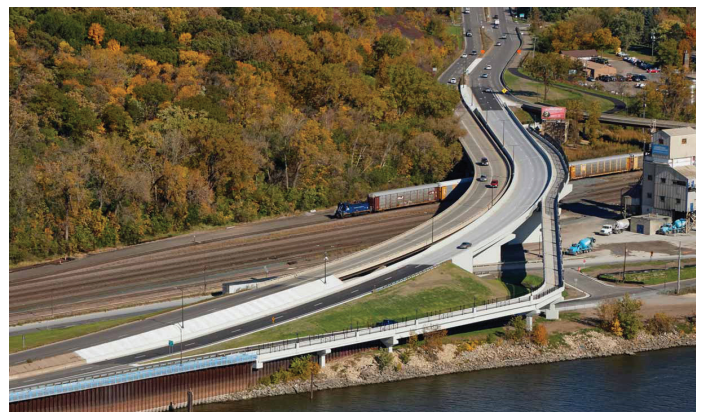
Figure 2.2 SMRT Warner Road Bridge. (Photo: TKDA)
