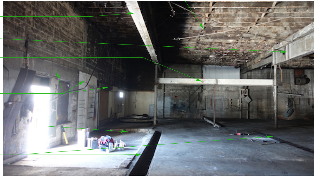
Toward North Wall
