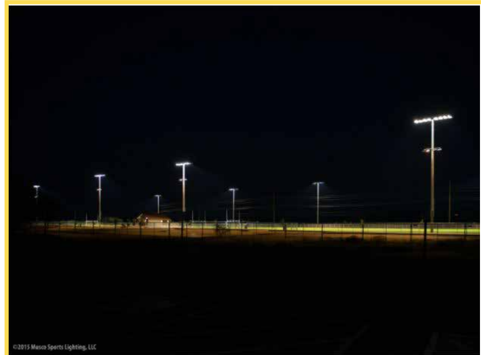
LED lighted soccer facility located adjacent to a residential neighborhood. Photo taken approximately 150' from field edge.
