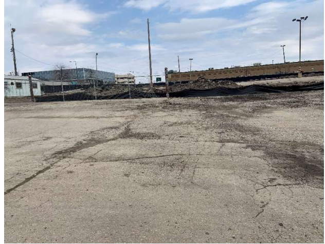
View from Subject site facing north
