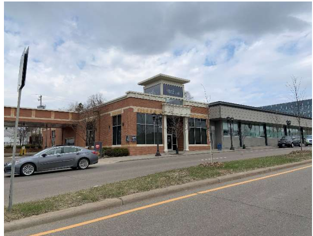
Typical commercial/retail uses east of Subject site
