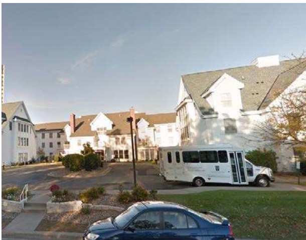
Assisted living facility north of Subject site
