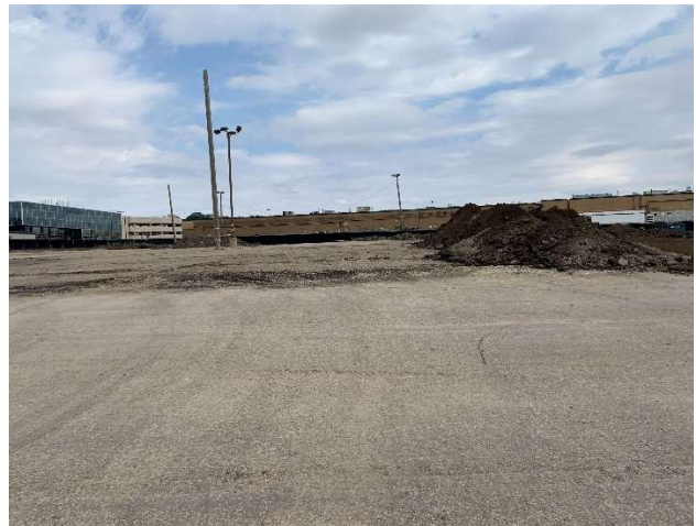
View from Subject site facing east
