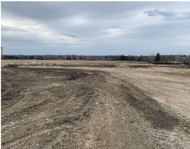
View from Subject site facing east
