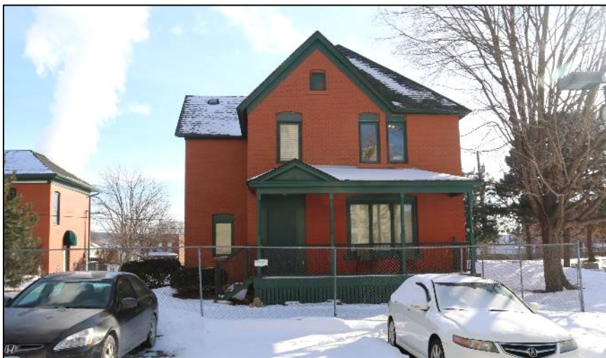
Figure 16. Joseph Walla House (RA-SPC-5311). Photographed facing south from Winslow Commons parking lot, February 2021.
