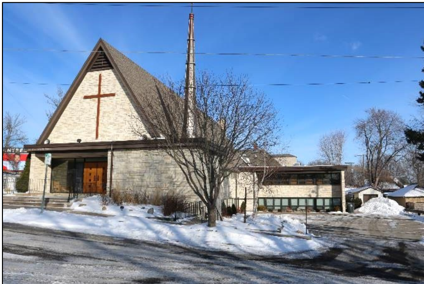
Figure 22. Saint Mark's Evangelical Lutheran Church (RA-SPC-8333). Photographed facing east from Ann Street, February 2021.
