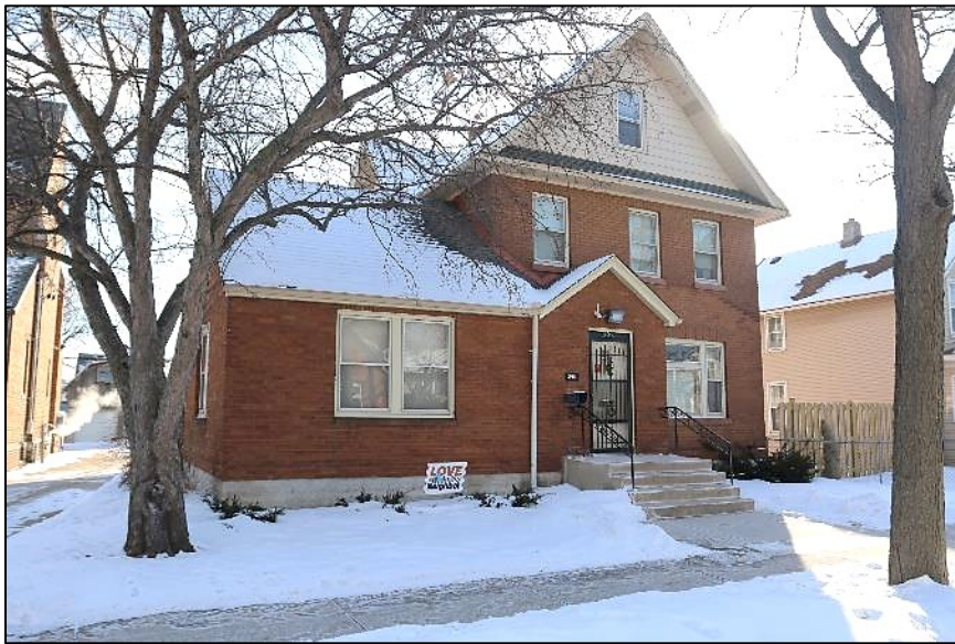
Figure 12. Saint Stanislaus Rectory (RA-SPC-3806). Photographed facing south on West Superior Street, February 2021.
