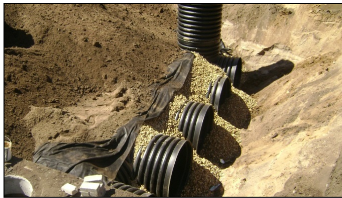
Photo 5-1: St. Albans 48" Perforated HDPE Installation
