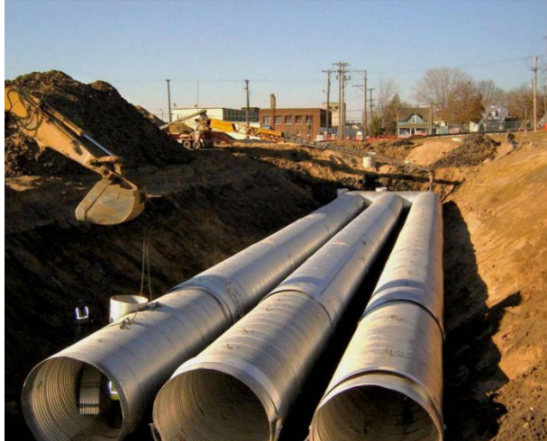
Photo 4-1: Underground Infiltration Chamber (Facing West)
