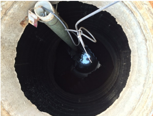
Photo 2-1: Infiltration Gallery Level Monitoring Enclosure
